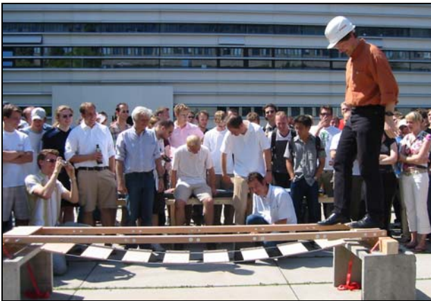
Figure 6: Student Project "Bridge in the Bag" – Testing in front of student audience
