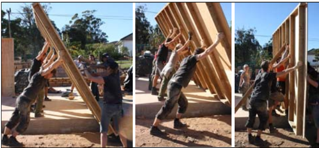
Figure 16: Design Project “Kindergarten Raithby” – Student team erecting a timber frame wall
