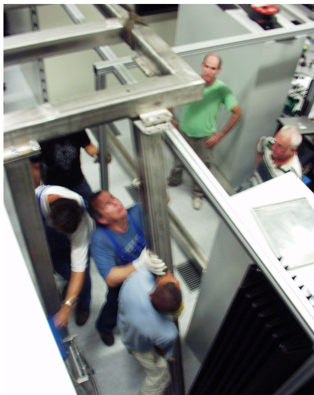
Figure A.5: During the construction laser work has to stop, so speed is of the essence.
