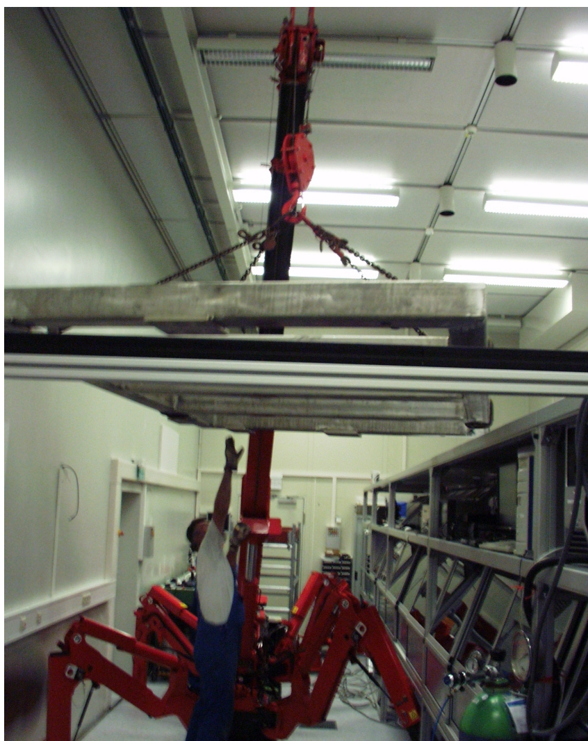
Figure A.2: Lifting a few hundred kilogram of steel frame above a sensitive high-power laser system.
