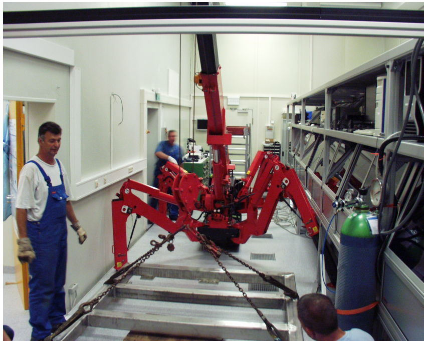
Figure A.1: The crane is ready to install the beamline in the cleanroom.
