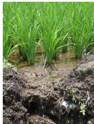
Figure 8: Water outlet to control the height of standing irrigation water.
