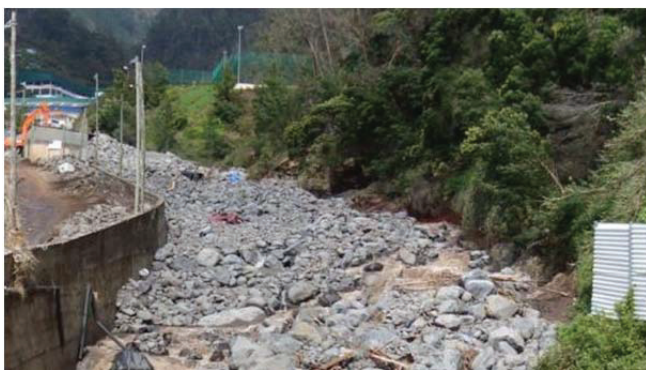
Fig. 1: A debris flow blocked a channel with huge boulders and entrained cars.
