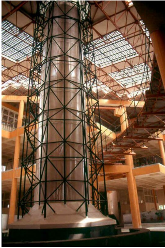
Fig. 10.0 Wind Tower and BIPV
