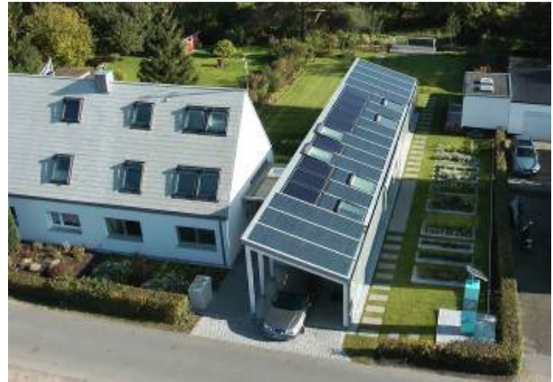
Figure 7: Photovoltaic modules and solar thermal collectors on the roof of the extension
