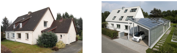
Figure 5: The LichtAktiv Haus before and after climate renovation
