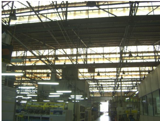
Figure 3: HDR image in Industry B - task illumination installed on a height closer to the workers' visual field.
