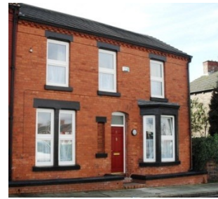
Figure 1: Terraced house after refurbishment.
