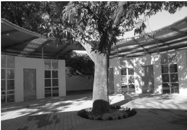
Figure 6: Sash windows, double roofing and shade maximize natural ventilation and lighting
