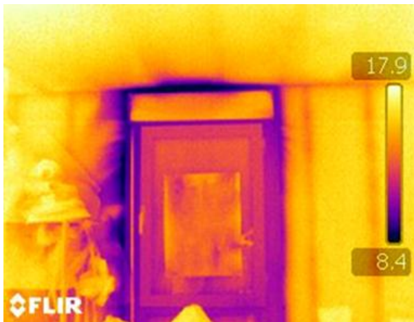
Figure 5. Thermographic image of RA3 type D dwelling
