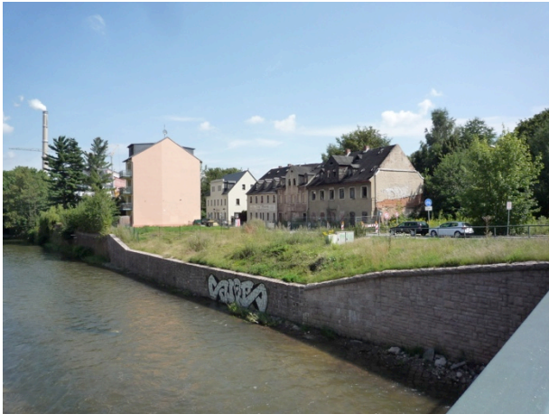
Image 5: Site in Hauboldstraße, Chemnitz, 2013 before
