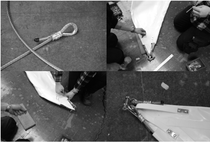
Figure 7.6: Assembling of the edge cables
