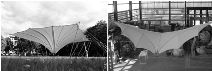
Figure 3.25: Hybrid tensile structures with integrated elastic members (left [LK12]; right [Off10])
