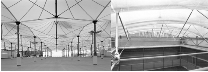
Figure 3.26: Hybrid tensile structures with external elastic members (left [Koc04]; right [Sei08])
