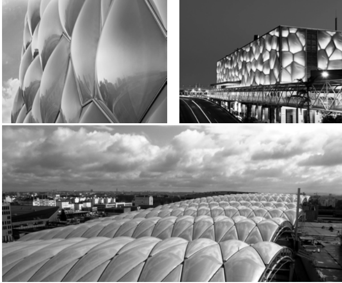
Figure 4.5: Examples for ETFE cushions; top: Casino Macao; bottom: Lyon Confluence (copyright: Seele Cover GmbH)
