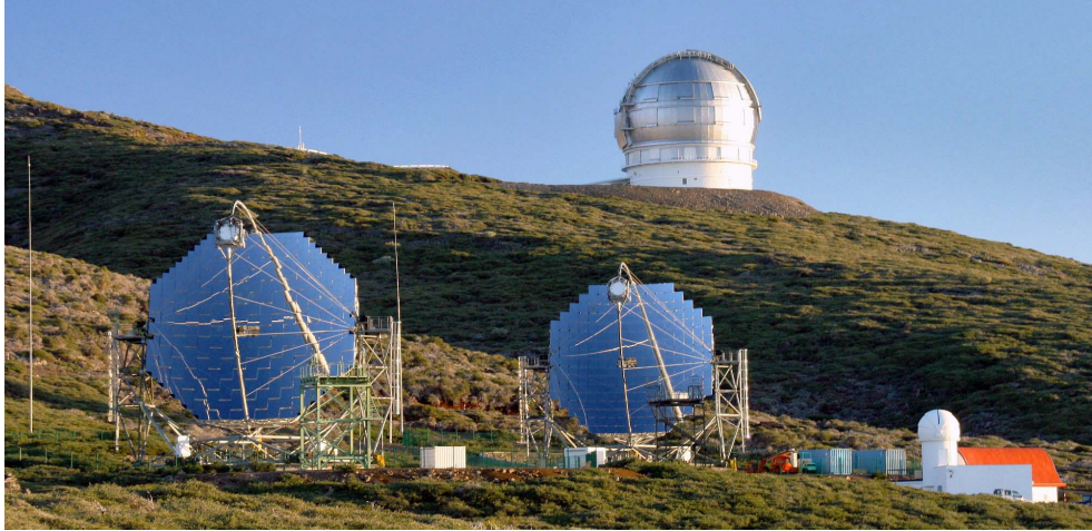
Figure 3.8: The MAGIC telescopes on top of the Roque de los Muchachos on the Canary island la Palma. From left: MAGIC I, MAGIC II and the LIDAR tower on top of the counting house. The Gran Telescopio Canarias (GTC), with 10.4 m main mirror largest single optical telescope world-wide, can be seen in the background. Image: courtesy of Robert Wagner
