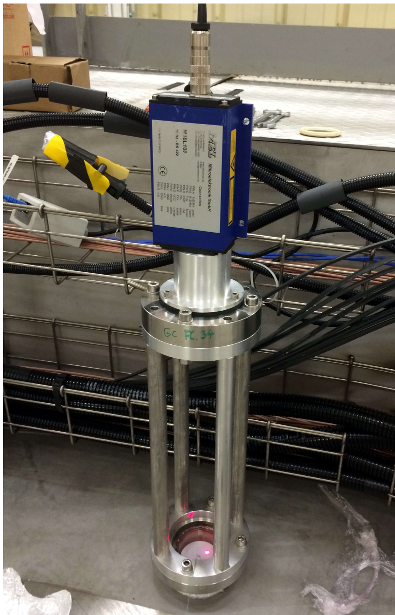
Figure 4.12: Installation and calibration of a laser sensor in Chooz. The laser sensor (blue box) is mounted in a adjustable bush. With screws, the surface perpendicular to the laser path can be adjusted accurately. For calibration, the laser flange with the adjustable bush is mounted to a solid and rigid extension. A dummy PTFE floater connected to a fishing line is lowered step by step into the laser guide tube. After each step, the laser path is readjusted until it is reaching the floater at the very bottom of the guide tube. Afterwards a PTFE floater without line was released into the guide tube and the laser flange was mounted directly onto the detector flange.
