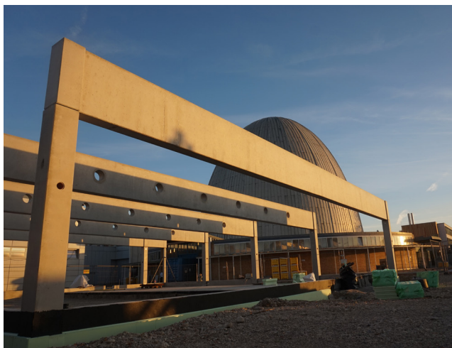
Figure 3: Construction of the storage hall for the radioprotection department.
