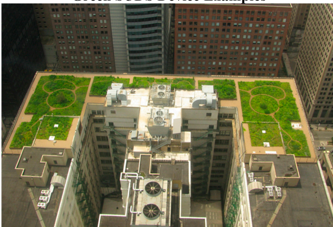
(a) Green Roof [1]
