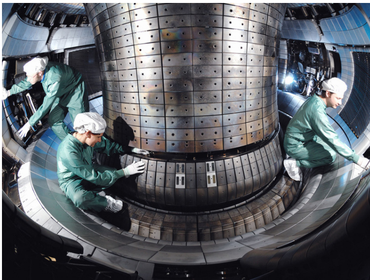
Figure 2.1.: The chamber of the ASDEX Upgrade tokamak during installation of the tungsten plasma facing components (source: IPP webpage)
