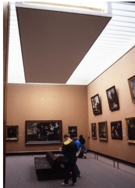
Figure 1.33 A perimeter luminance ceiling in the North Wing of the National Gallery, London. (Christopher Cuttle, Light for Art's Sake, p89).
