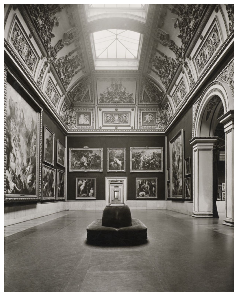
Figure 1.23 (right) A contemporary photo for gallery IX in the Alt Pinakothek, Munich, Germany. It shows the changes occurred to the laylight and the vault. ( https://en.wikipedia.org/wiki/Alte_Pinakothek )
