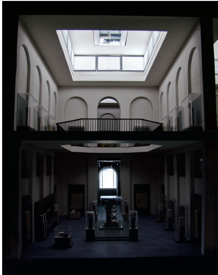
Figure 5.139 The light atmosphere in the Large Side Hall UF. The louvres of the diffuser-box system direct the light onto the upper parts of the walls and the ceiling. It creates a soft and diffuse atmosphere that will support the artificial light of showcases. The systems is glare free and do not create veiling reflection on the showcases.
