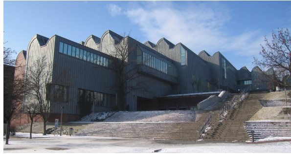
Figure 1.34 The Polar-oriented skylights on the top of Ludwig museum characterize the building. (Ludwig Museum, Cologne, Germany).
