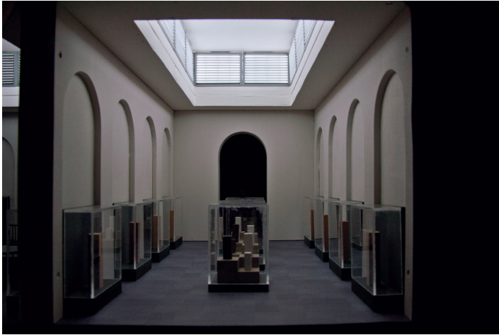
Figure 5.144 The light atmosphere in the Small Side Hall UF. The louvres of the diffuser-box system creates a soft and diffuse atmosphere that will support the artificial light of showcases. Compare the result with (Figure 5.16 and Figure 5.48).
