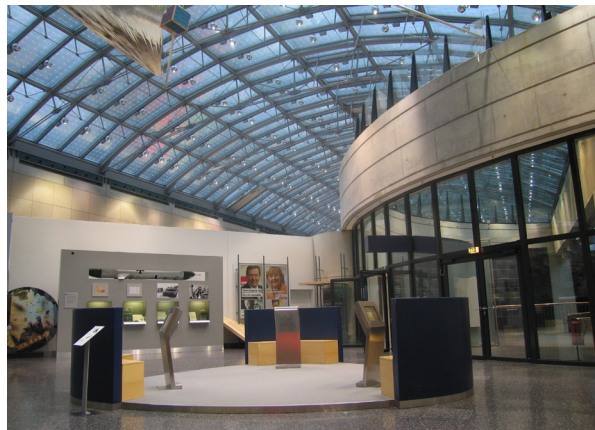
Figure 1.27 Interior view of the glass roof. The photo was taken during the afternoon time and the sky was totally covered with clouds and the artificial light was turned on. The translucent connection to the bluish light of the sky outside adds a natural feeling to the space. (House of History Museum, Bonn, Germany).
