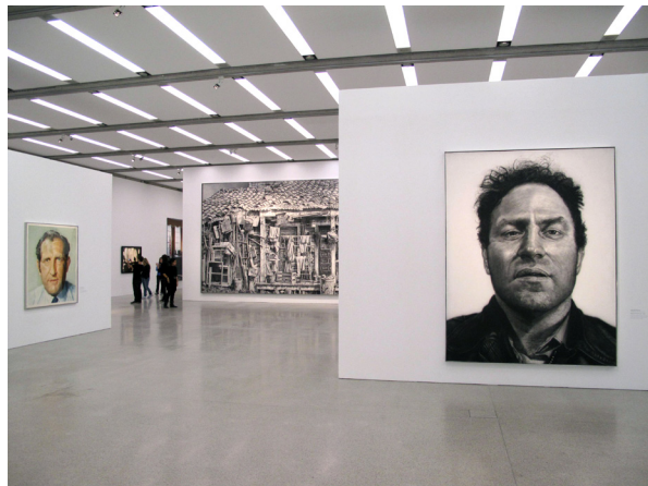
Figure 1.59 An array of diffuse rectangular luminaire can be more efficient than overall diffuse ceiling. (MoMA, Museum of Modern Art, Vienna, Austria).
