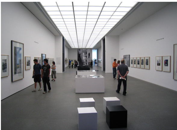
Figure 1.57 Overall luminous ceilings. (Architekturmuseum der TU München – Home in Pinakothek der Moderne, Munich, Germany)
