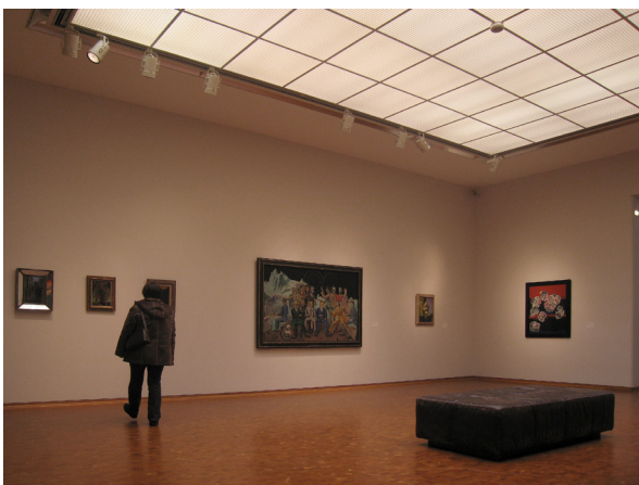
Figure 1.61 An artificial lighting louvre ceiling as general illumination and spotlight on tracks to softly highlight the exhibits. The ceiling is fitted as well with wall-washer in case the walls need to be brightly illuminated. The illumination level is lowered for the sake of the painting conservation. (Ludwig Museum, Cologne, Germany).
