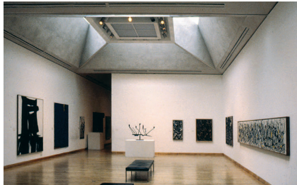
Figure 1.46 A baffles system that direct light more to the walls. The extension of The Tate Gallery, London, 1979. (Christopher Cuttle, Light for Art's Sake, p109).
