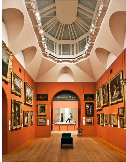
Figure 1.19 (left) Dulwich Picture Gallery, London, UK. A photo from (1974) showing the modification occurred to the skylight by glazing in the sloping roof elements. ( http://www.dulwichpicturegallery.org.uk/about/our-architecture/ ).
