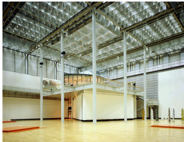
Figure 1.42 The daylight grid louvres ceiling directs the luminance of the glass roof inside the main hall. Art Museum Wolfsburg, Germany. (with permission of Bartenbach GmbH).
