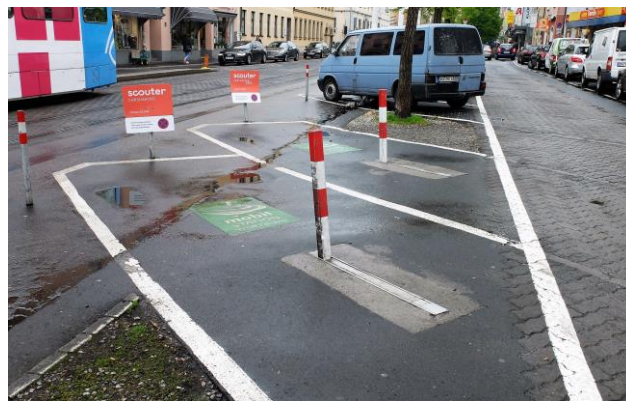
Figure 16: Collapsible bollards at the station Juliuspromenade (own picture)
