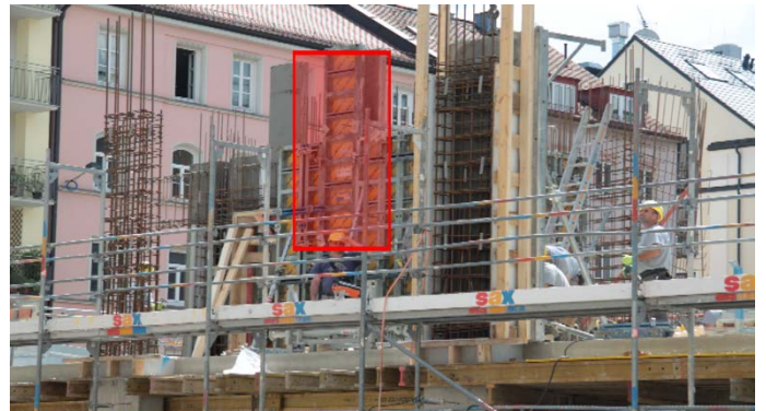
Figure 5: Detected bounding box for formwork elements on a photography of a construction site.
