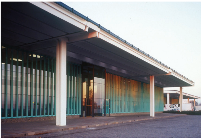
Fig. B.3: Isocell U70, application in industrial building in Turate (Como, I, 1982), architect Angelo Mangiarotti (Matthias Bräm)
