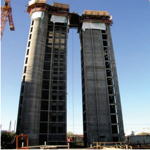
Fig. C.9: Stairwell/elevators cores built using sliding formwork (Gleitbau GmbH, 2006)
