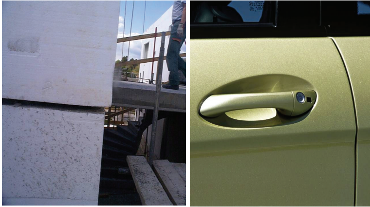
Fig. E.1: The lack of experience with the new and stricter tolerance requirements led to extra and unnecessary work at the building site (LANDIN) 2004. The manufacturing industry can be a source of inspiration to the building industry through its far stricter tolerance requirements.
