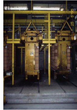
Fig. B.15: run-dry station
