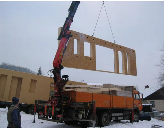
Fig. I.8: Panel construction of a (timber) building
