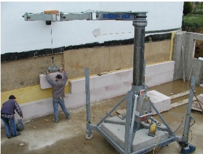
Fig. B.32: Layher balancer with mechanical stone gripper
