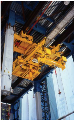
Fig. I.13: column placing system
