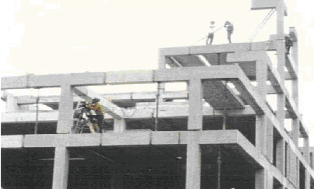
Fig. B.6: Installation of Componoform integrated joint precast concrete components
