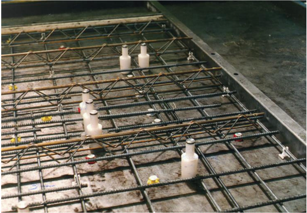
Fig. F.5: Screw sockets and sparings
