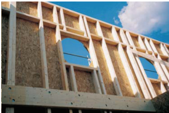
Fig. I.6: Ribbed wall construction (Informationsdienst Holz, 2000)
