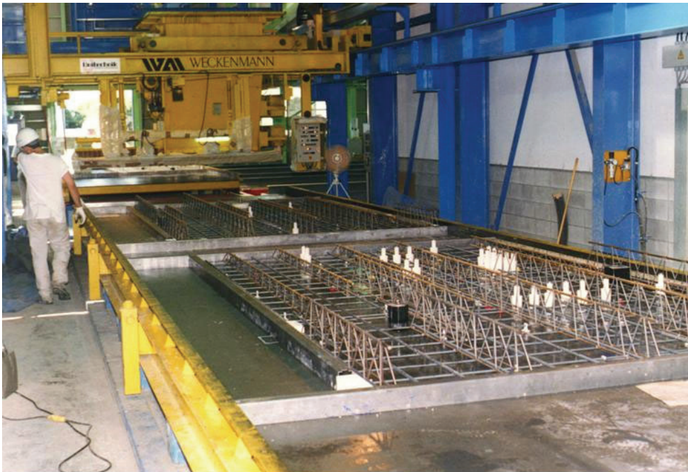
Fig. F.6: Pallet in concreting station
