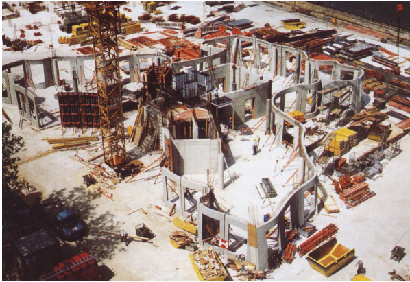
Fig. F.13: first floor: just-in-time assembly of the elements
