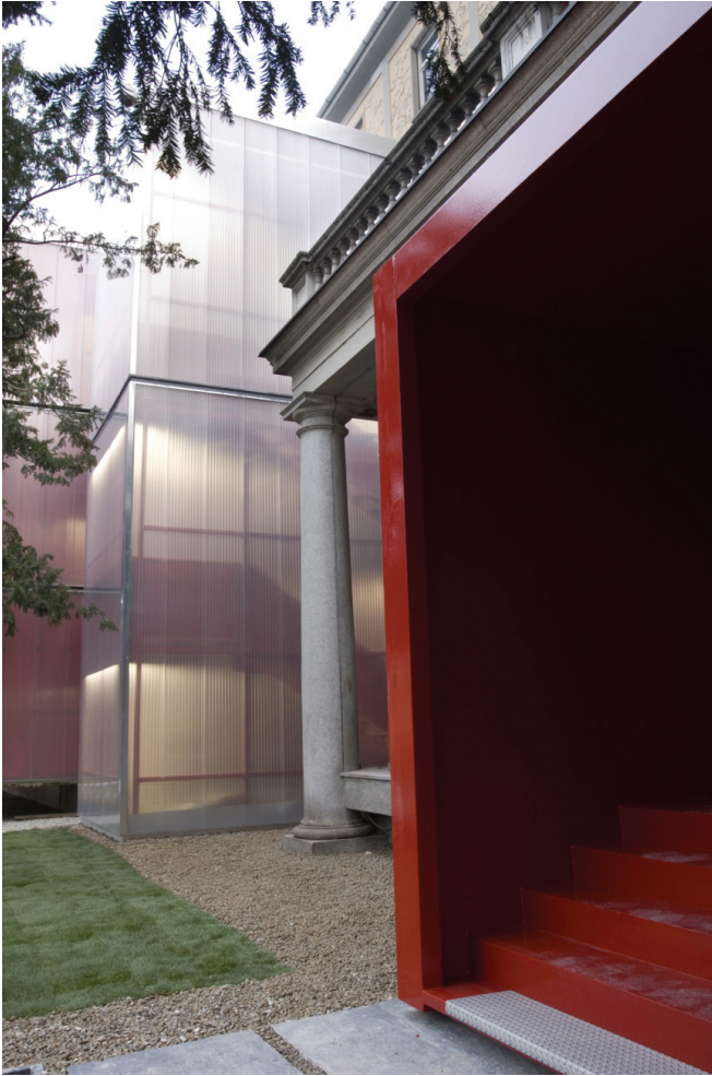
Fig. C.15: Research Campus Point in Lecco: New temporary offices integrated to the existing building (NORLIGHT, 2007)
