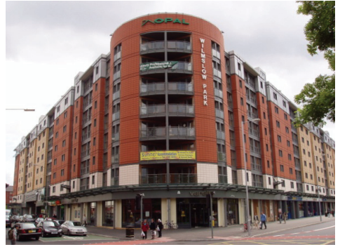
Fig. E.4: Mixed commercial-residential development in Manchester using 1400 modules on a steel-composite podium structure for the ground floor and basement
