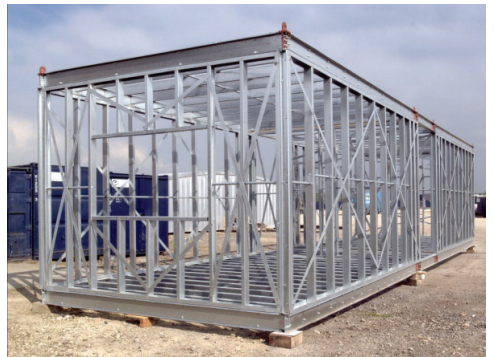
Fig. E.10: Corner-supported module (Kingspan Off-site)
