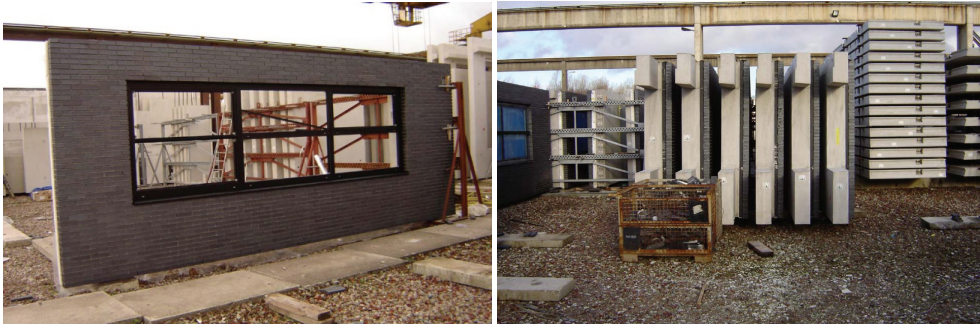
Fig. G.3: Mounting of casings and glazing; storage of the units
