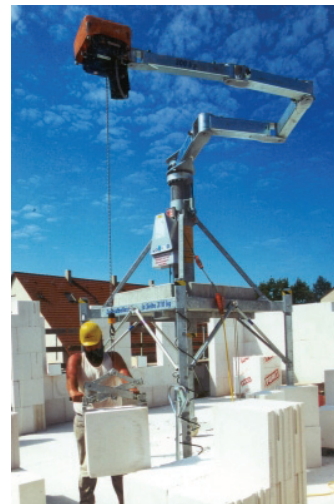
Fig. B.33: Scissor type gripper on sacra balancer
