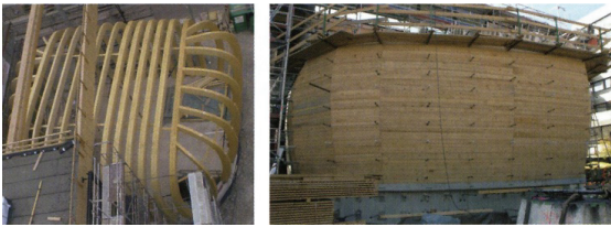
Fig. F.23: assembly of the wood structure
