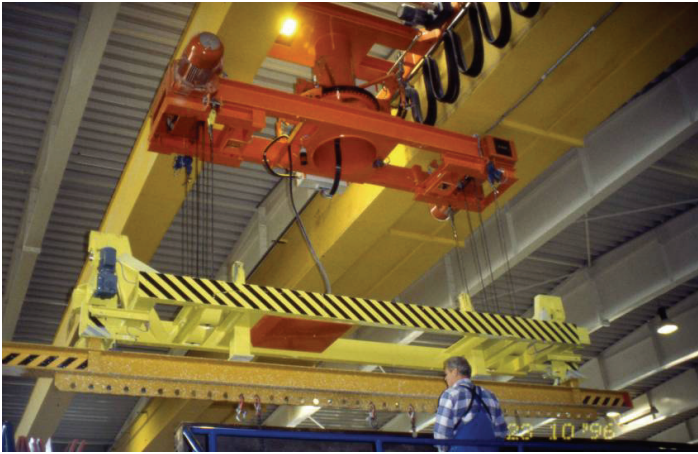
Fig. B.20: factory logistics indoor
