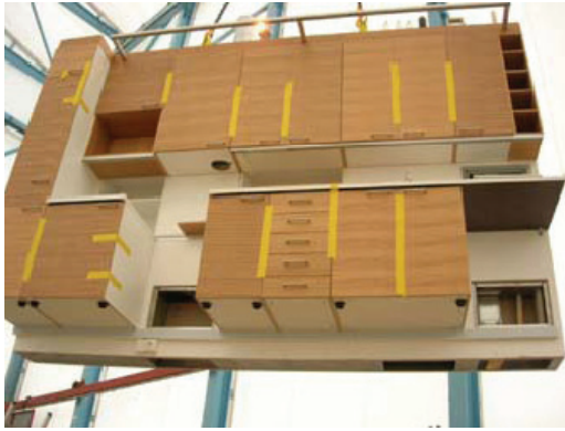
Fig. I.8: assembly of prefabricated wall components in on-site assembly hall
