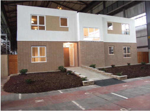
Fig. E.11: Demonstration building using mixed panel and modular construction
