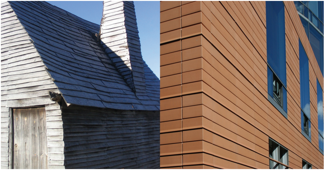
Fig. E.1: Slight variations of façade shingles in vernacular buildings are rather difficult to replicate with today's industrialised production methods.
