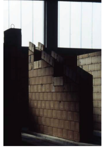
Fig. B.29: final brickwork panel product
