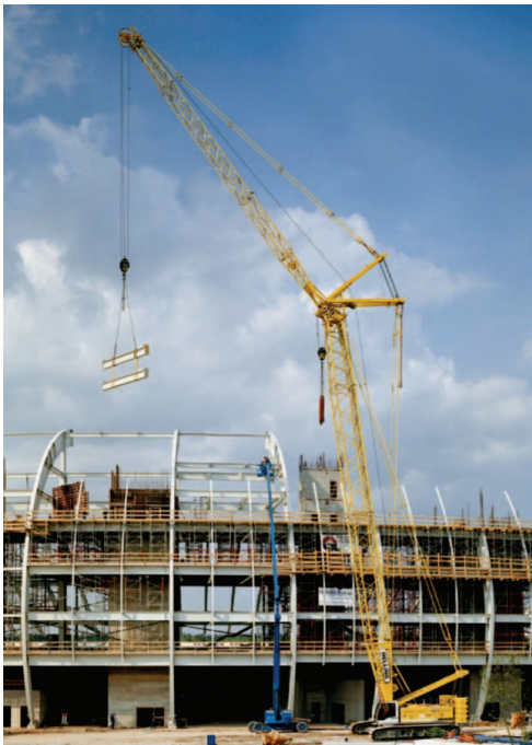
Fig. G.32: Assembly using a mobile crane (August Bammer, 2006)
