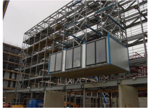
Fig. E.14: Steel framework supporting open sided modules- MOHO , Manchester (Yorkon)
