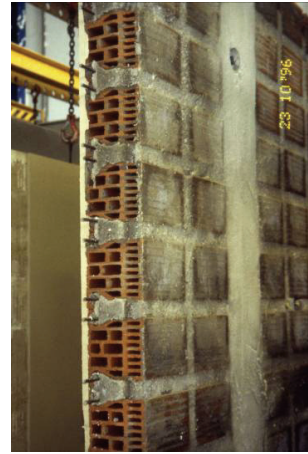
Fig. B.21: bare brickwork floor panel
