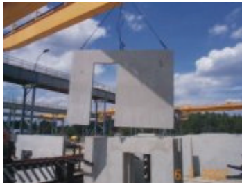
Fig. H.17: Bogucin Plant, Poland – basement walls
