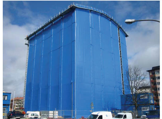
Fig. I.9: On-site factory of NCC Complete
