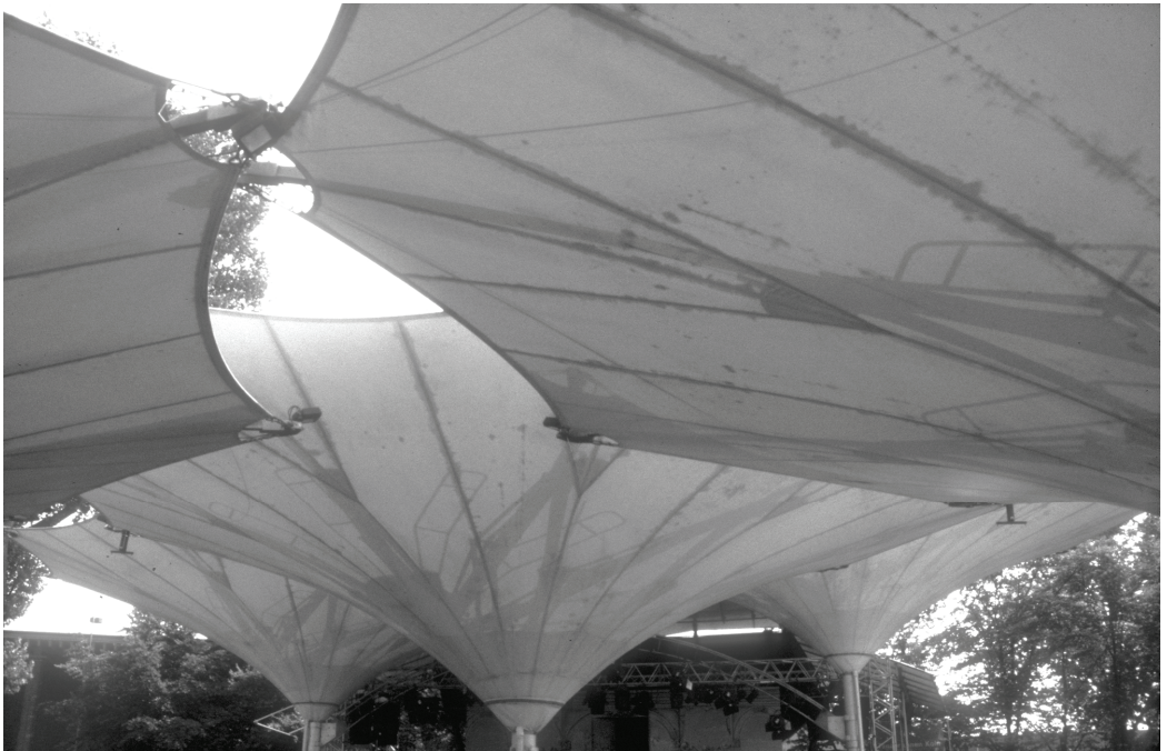
Fig. E.5: Tensile membranes are a good example of custom fabrication, supported by well-developed and integrated design and fabrication automation systems.
