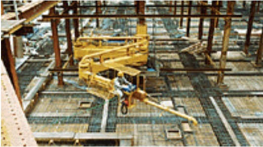
Fig. C.13: Concrete spreader (Takenaka Corp, 2006)
