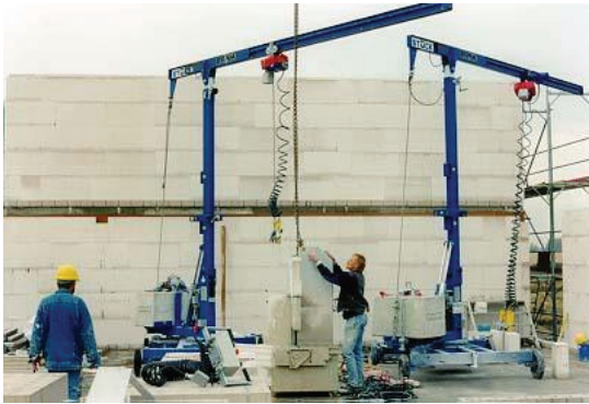
Fig. C.16: Offset rig for large-size bricks (Bilfinger+Berger AG, 1998)
