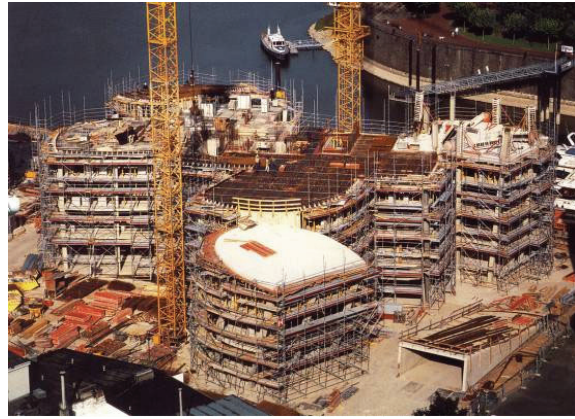
Fig. F.16: structural works House C
