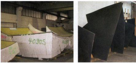
Fig. F.22: production of the glassfiber-concrete elements
