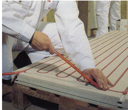
Fig. H.17: Board element with heating pipes
