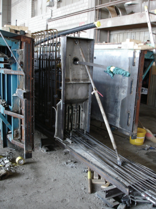
Fig. G.9: Prestressing strands in a stressedbed (Element AG)
