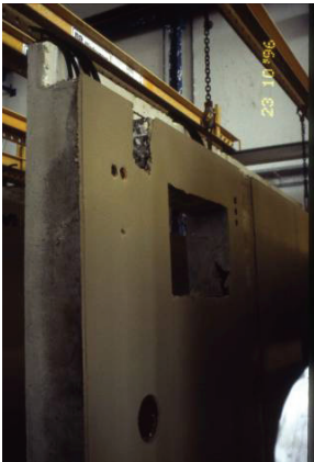
Fig. B.22: brickwork panel with plaster
