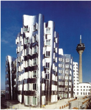
Fig. F.10: House B stainless steel facade
