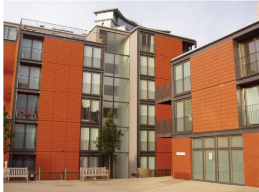
Fig. E.2: Completed mixed panel and modular project at Lillie Road, Fulham, London
