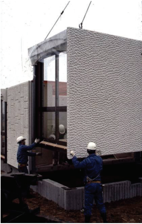
Fig. B.3: Installation of a PALC covered Misawa 3D module
