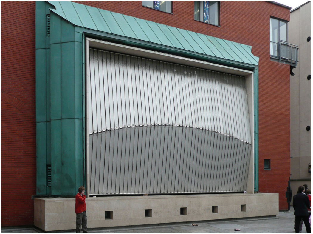
Fig. E.3: This gate in Dublin, Ireland, involves only a simple length variation of the individual aluminium elements. When open the bottom edge translates up vertically, and the gate forms into a complexly curved form.
