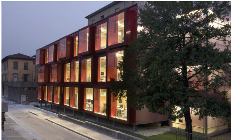
Fig. C.14: Research Campus Point in Lecco: The temporary office is a three storey construction built in front of the old hospital existing structure of Politecnico di Milano campus, in Lecco (NORLIGHT, 2007)
