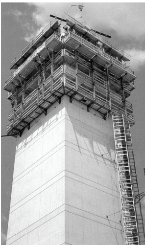
Fig. C.10: Self-climbing formwork, SCP (DOKA)
