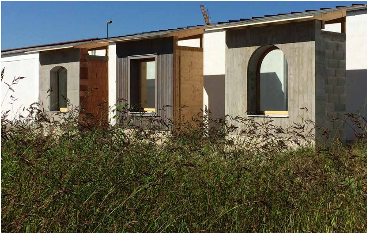
Image: Three façade models in thermal insulation masonry, solid wood and lightweight concrete construction (Photo: Tilmann Jarmer)
