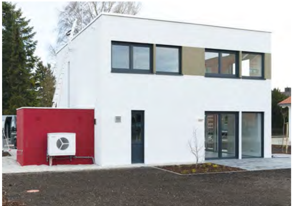
■ Dynahaus building finished in December 2014.
