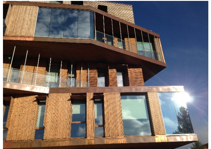
Figure 2. A six-storey wooden building of solid cross-laminated timber walls and slabs and articulated topography of the facade, NINA Trondheim.
