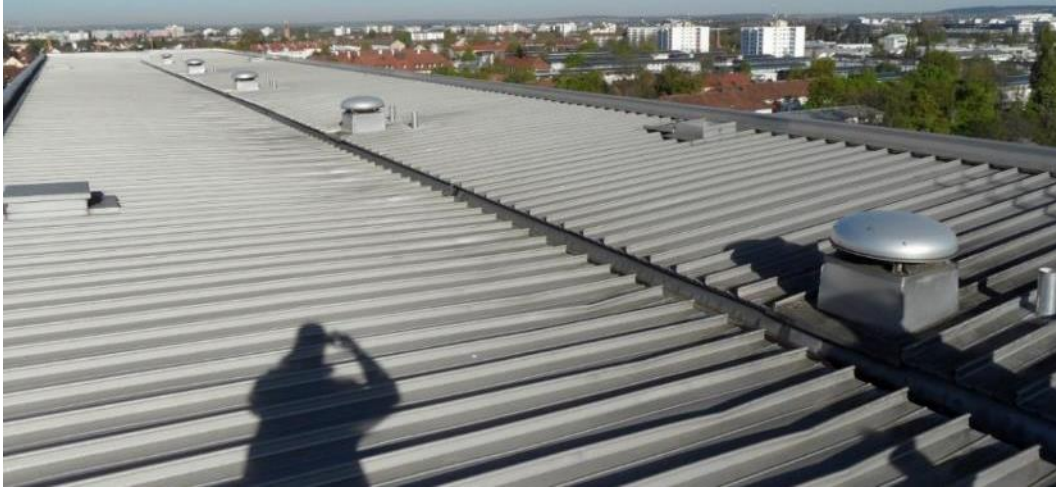
Figure 31: Flat tin roof of building 1 (west side)
