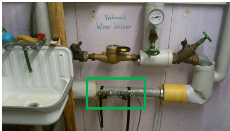
Figure 34: Acquisition of hot water consumption profiles by means of an ultrasonic clamp-on flow meter at the cold water inlet of a hot water storage
