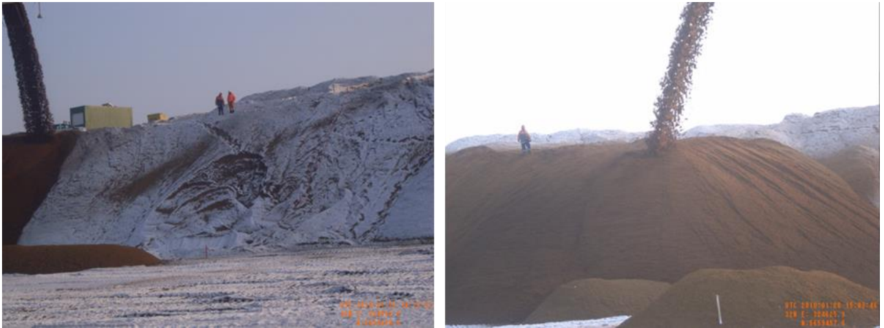
Figure A.12.3: Dumping above hydrostatic measuring line and measurement gauge HSP-LS1, printed with permission from RWE Power AG
