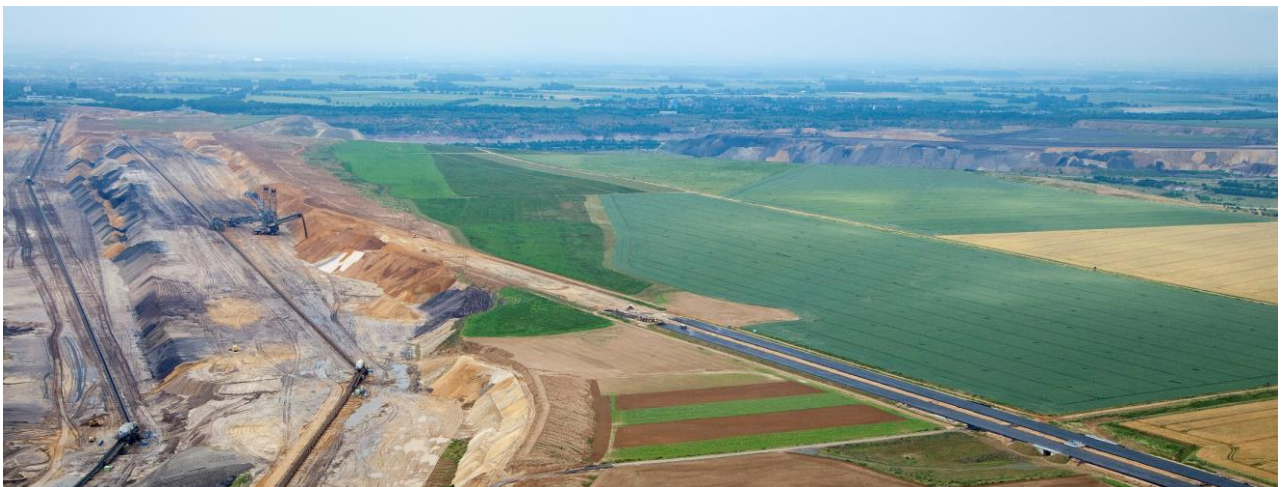
Figure 1.1: Construction of highway A44n on Garzweiler open cast mining dump near Cologne (Germany), printed with permission of RWE Power AG
