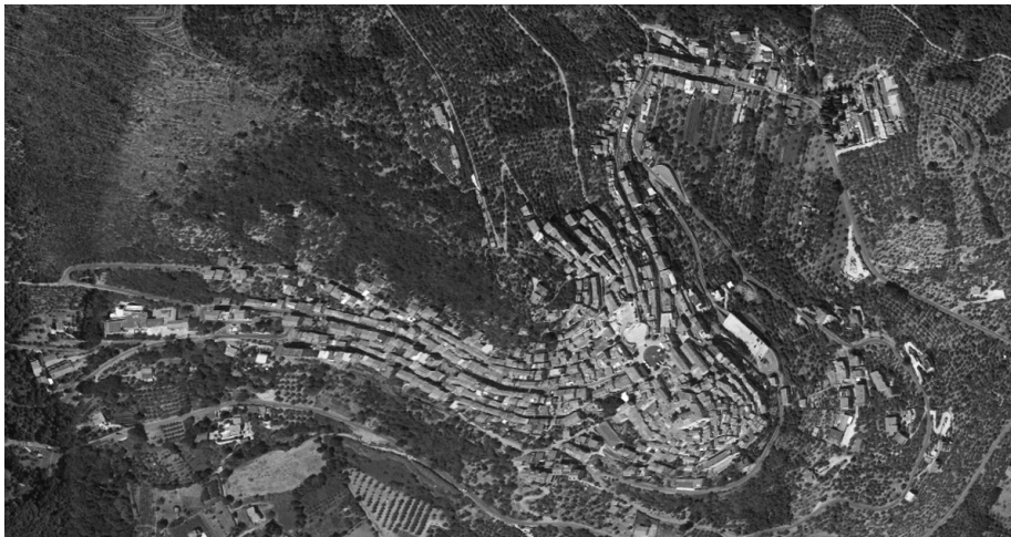
Fig 9.8 Aerial view of Roccagorga (source: Google Earth)
