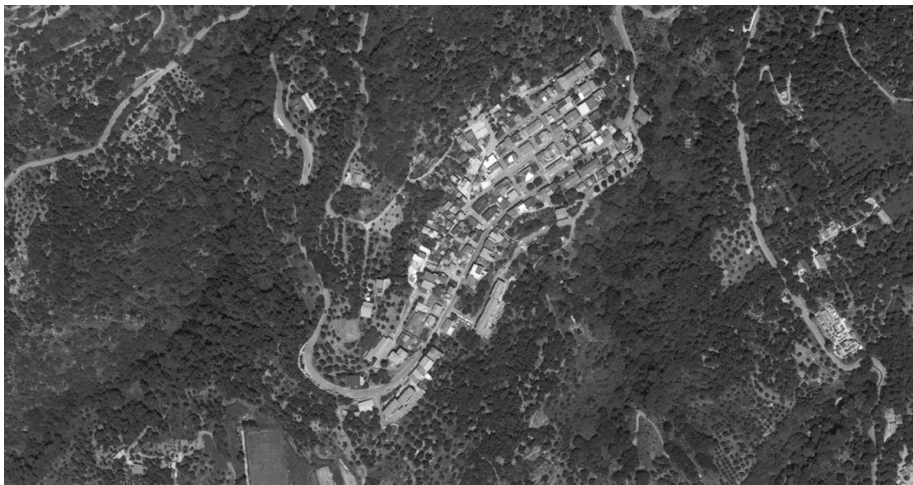
Fig 9.4 Aerial view of Sant'Alessio (source: Google Earth)
