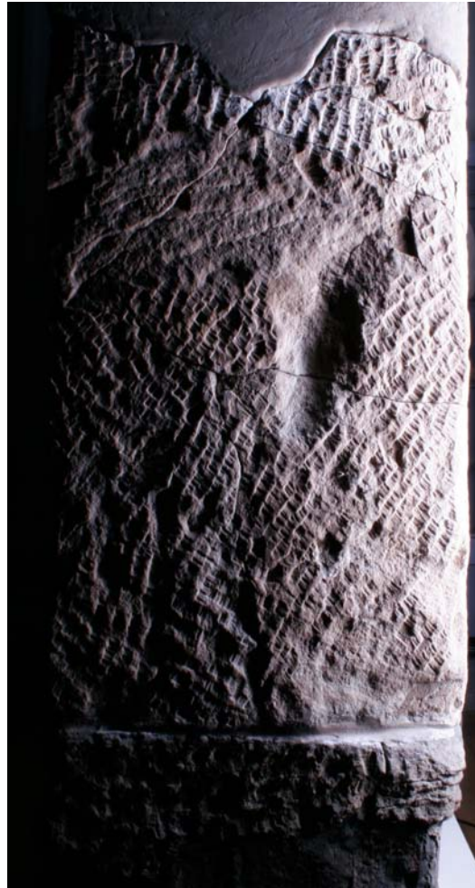
Figure 19 The 'rough tooled' back in raking light
