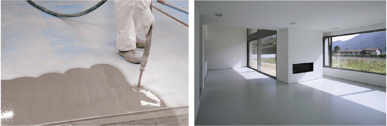
Figure 6: Application of self-levelling underlayments (SLUs) [53]. Reprinted with permission.
