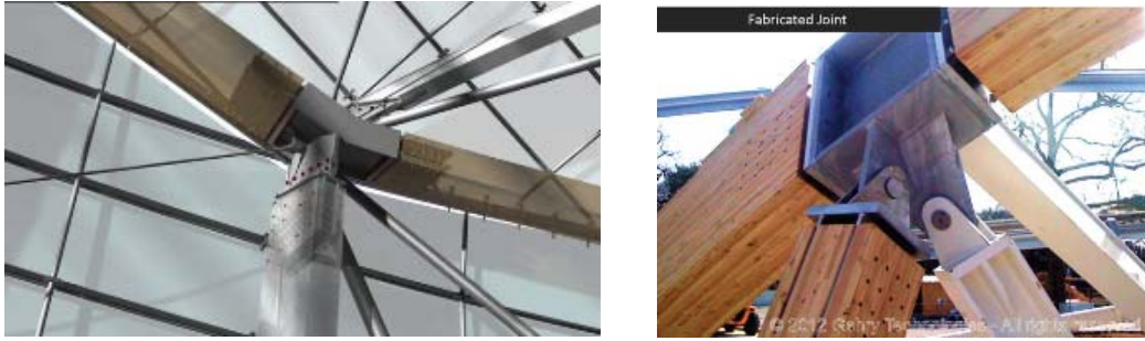
Figure 15: Joint - 3D modelling and fabricated (Gehry Technologies)
