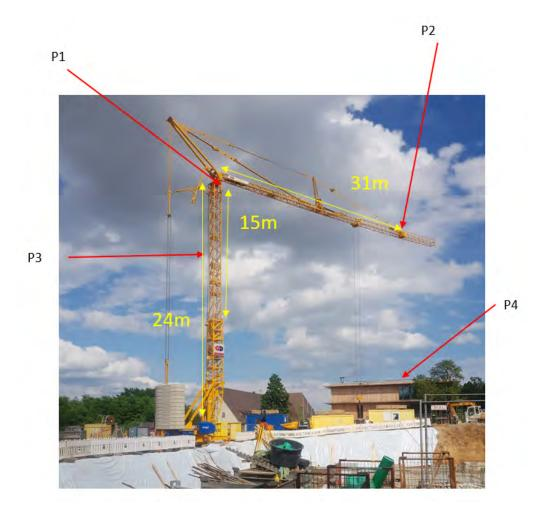
Figure 5.10: Positions of crane cameras
