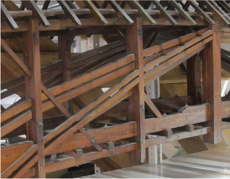
Fig. 7 Original model of the ‘Trogen bridge’ made by the Grubenmann brothers (around 1745–1755), Grubenmannmuseum, Teufen, Switzerland. (Image: Dirk Bühler)
