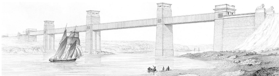
Fig. 1 Britannia bridge across the Menai Strait in North Wales. (Image: Clark 1850, Plate VI)
