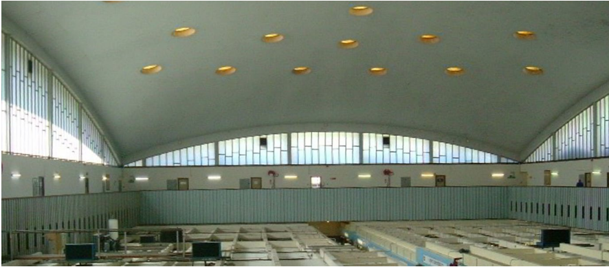
Fig. 13 Reinforced-concrete shell roof, Smithfield Poultry Market, London, 1963. (Image: Bill Addis)
