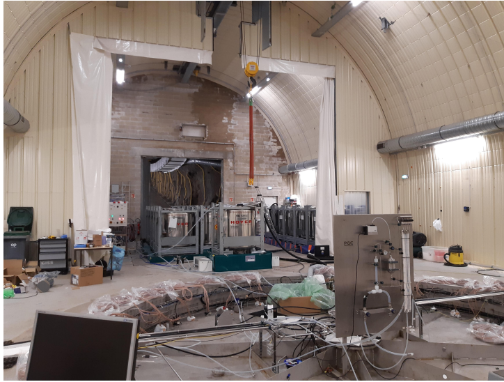
Figure 10.7: Overview of the emptying operation. XRS, IBCs and pumps are visible.
