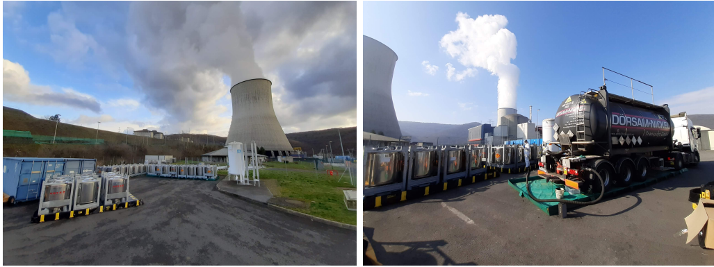
Figure 10.8: left : Full IBCs in the storage area. right : Liquid transfer from the IBCs to a truck.
