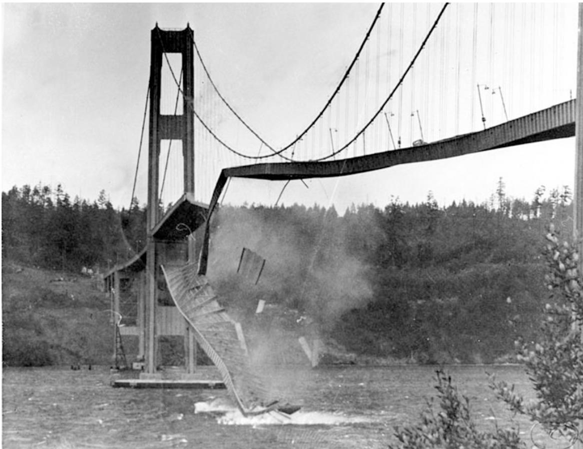
Figure 1.1 | Suspended Tacoma Narrows Bridge in November 1940.
