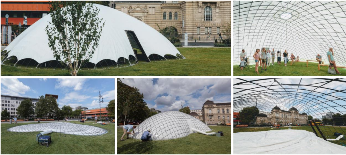
Figure 45 SheltAir Pavilion, erected using inflation: a) Outside view, b) Interior view, c) Flat assembly state, d) Inflation using cushion for erection, e) fixed and supported grid, the cushion is removed. (Quinn, 2018a)
