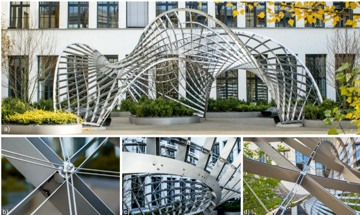
Figure 105 The inside\Out pavilion at TUM Campus, Munich: a) View of the pavilion, b) Node detail, c) Free edge beam and c) Singularity (Photos: Felix Noe)
