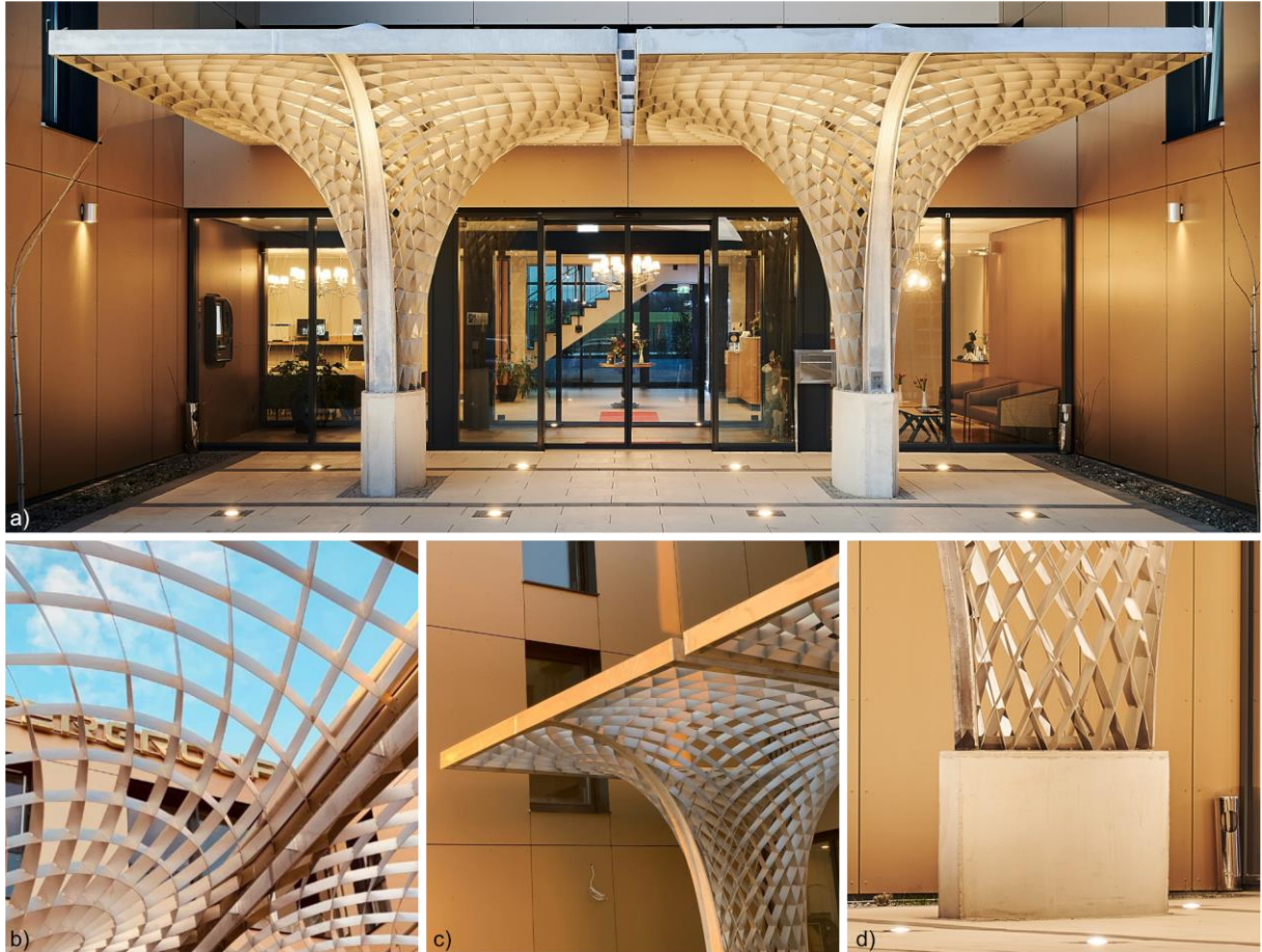
Figure 108 The Hotel Intergroup canopy (before membrane assembly): a) Front view b, c) Edge beam detail, d) Concrete foundation
