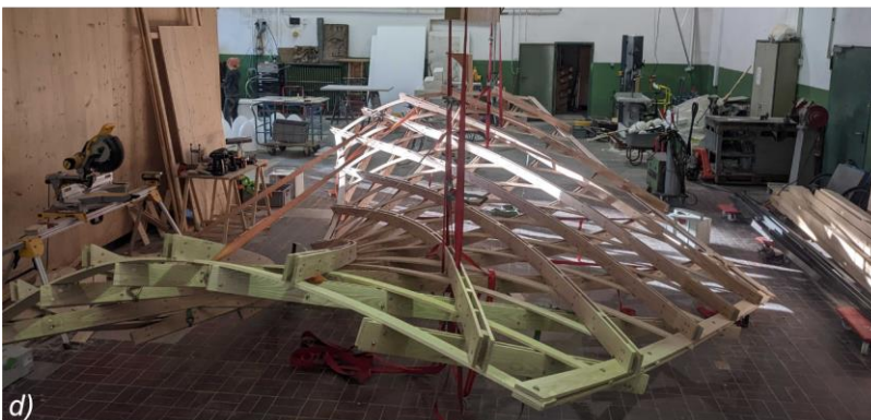
Figure 114 The Asymptotic Geodesic Timber Vault: a) View of the structure without cladding, b) Top view, (asymptotic curve set), c) Detailed view of the grid (web), including asymptotic (“upright”) lamellas and geodesics (“flat”) lamellas d) Shaping the grid structure from flat to spatial. e) Prefabricated curved, doubled lamellas.
