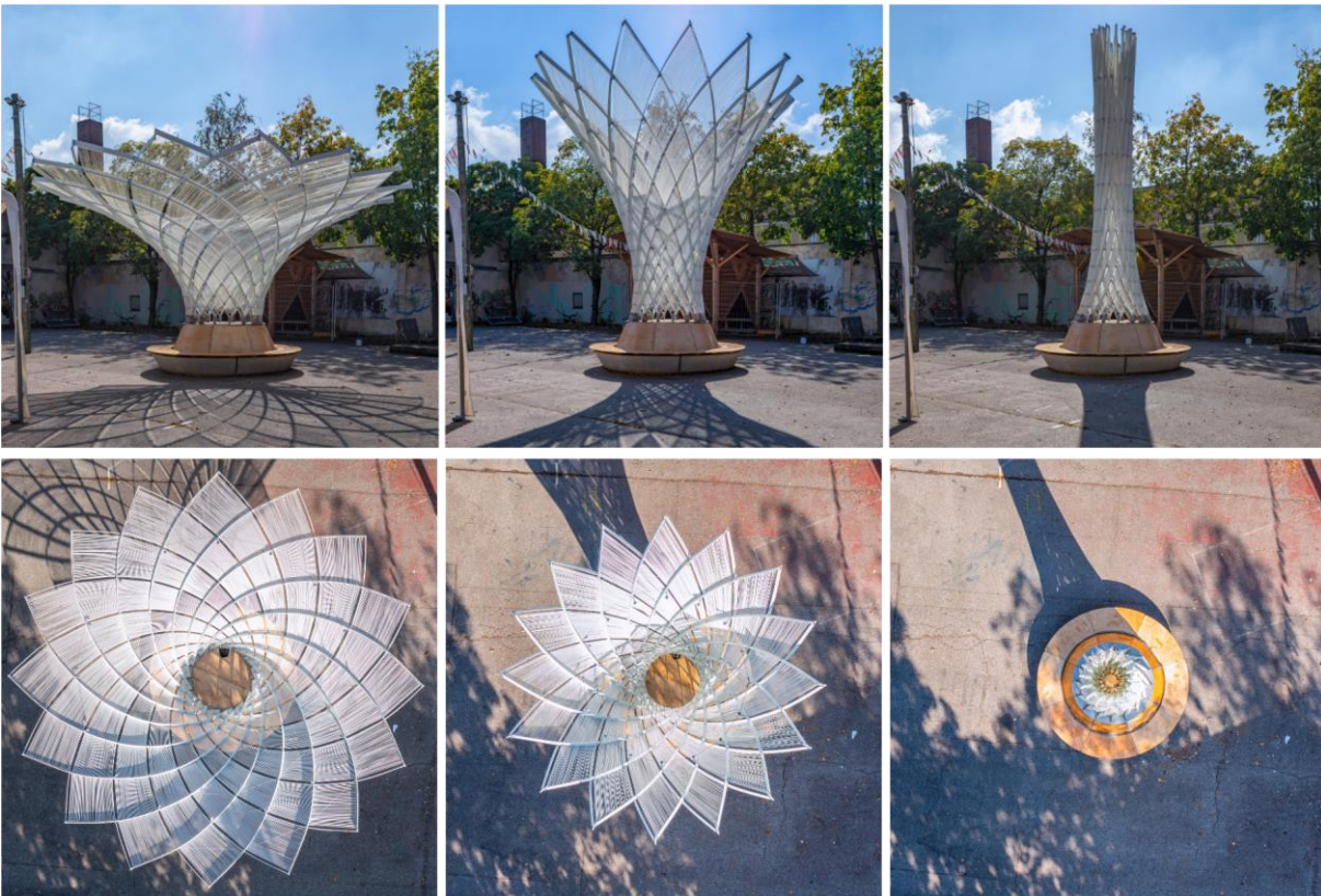
Figure 115 Side- and topview from open (left) to closed state (right) of the “Kinetic Umbrella” at the Kreativquartier Munich. (Photos: Martina Schikore)
