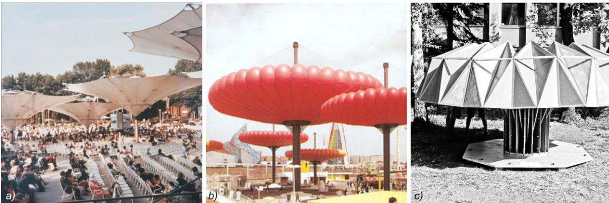
Figure 116 Various Umbrellas utilizing different mechanical approaches: a) Umbrellas by Frei Otto at the Bundesgartenschau Köln 1971, Photo: Atelier Frei Otto Warmbronn b) Inflatable Umbrellas World Expo, Osaka 1970 (Blümel, 1972) c) Umbrella Study using origami folding (Jaksch & Sedlak, 2011)
