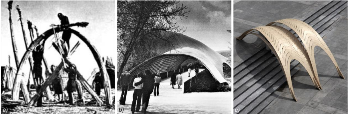
Figure 38 Built bending-active Structures, designed using varying approaches: a) Mudhif house in Southern Iraq. The building technic is still used today (Lienhard, 2014, p. 53), the design is “behavior”-based, b) Multihalle Mannheim build 1974, designed using a geometry based approach (Burkhardt & Bächer, 1978), c) The AA/ETH-Pavilion build 2011 at the ETH, designed using the integral approach (D’Acunto & Kotnik, 2013)
