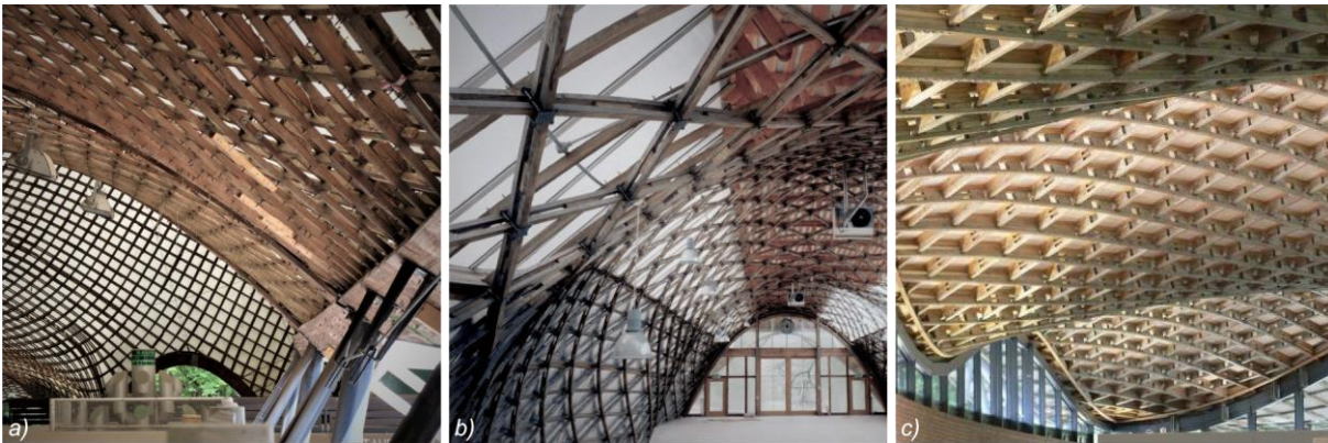
Figure 42 Strained timber Gridshells: a) Multihalle Mannheim (GER, 1974, Architect: Mutchler&Partner, Engineering: Ove-Arup&Partner and Frei Otto), b) Weald and Downland Museum (Johnson, 2002) c) The Savill Building (b, c: Du Peloux de Saint Romain, 2017).
