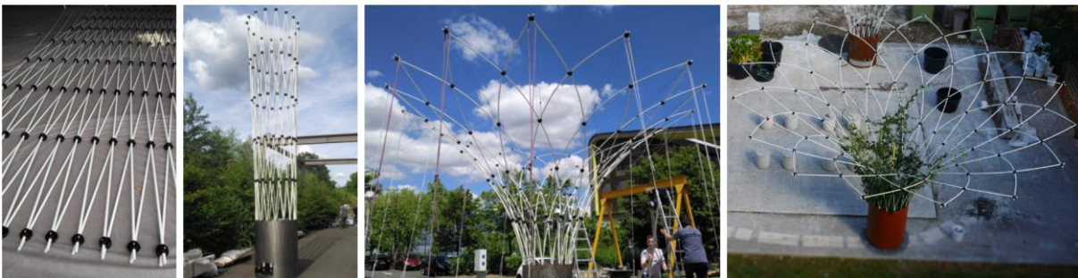
Figure 46 Funnel shaped gridshell for the support of climbing plants (ENPC, 2020)
