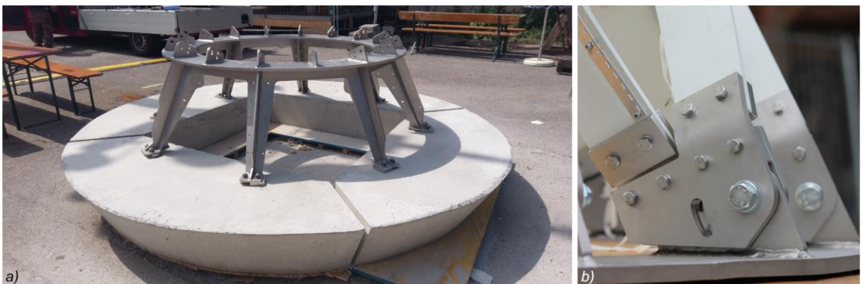
Figure 123 Base of the Kinetic Umbrella: a) Concrete bodies and steels support, b) Grid support detail (hinge)
