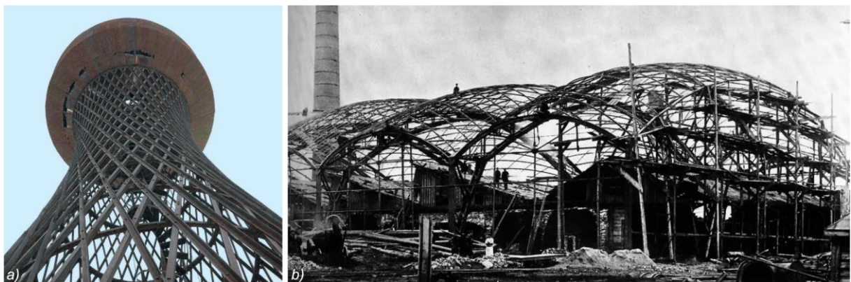
Figure 41 Steel gridshells from Vladimir Šuchov: a) Hyperboloid shaped Water Tower in Niznij Novgotod with twisted L-profiles (Beckh, 2012) b) Workshop in Vyksa (RU 1897) (Picture in public domain, taken from MARCH, 2020)
