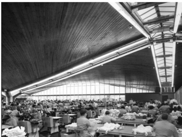
Figure 18: Roof structure of the “Silhouette Corset Factory, Market Drayton” made from symmetric timber HP-shells [31]
