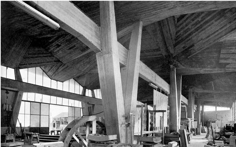
Figure 4.7: Stabilimento Raffa in Pietrasanta (1956). Interior view (Musmeci 1960, pp. 713).
