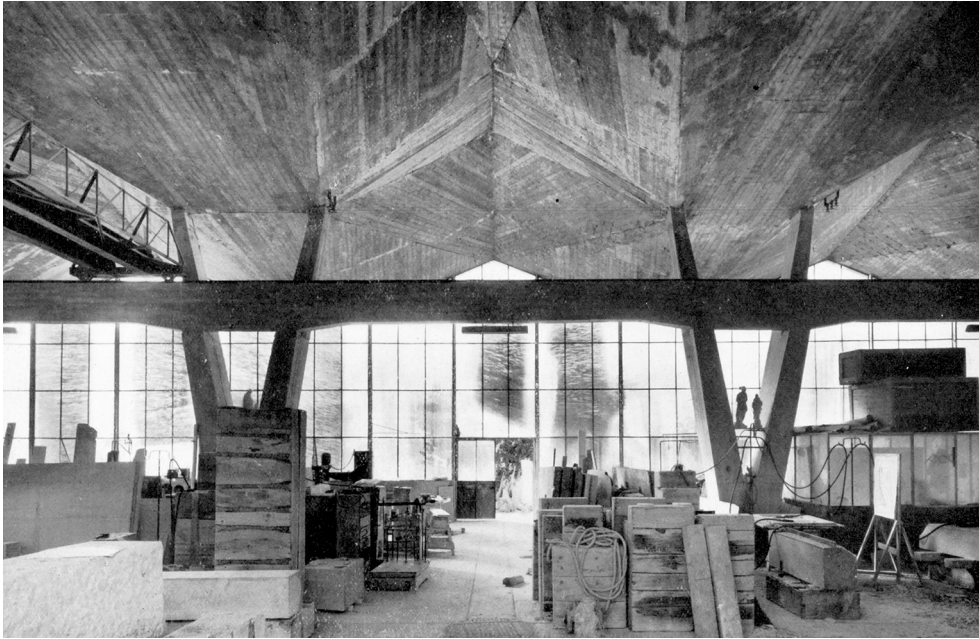
Figure 4.6: Stabilimento Raffa in Pietrasanta (1956). Interior view (Musmeci 1960, pp. 712).
