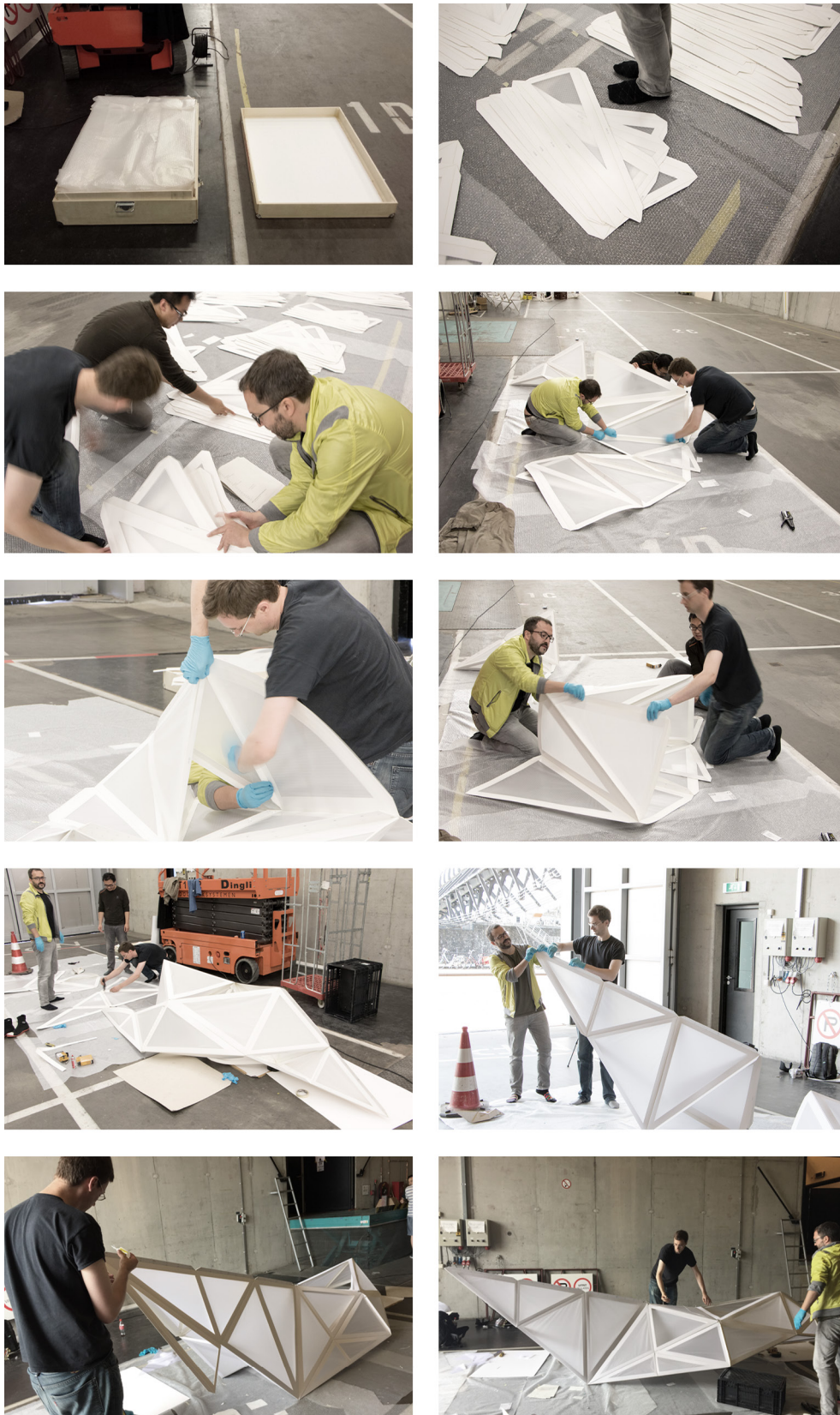
Figure 16.10: On-site assembly process of the foldKITE.
