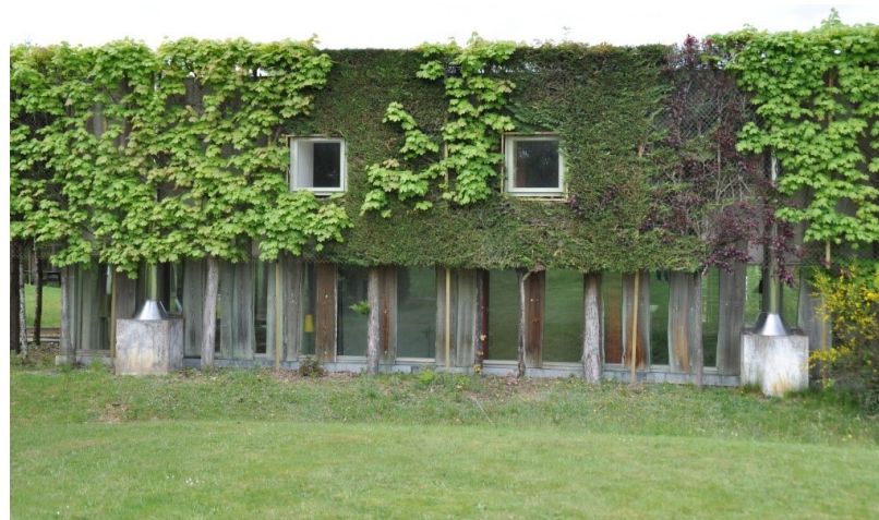
Figure 13. A tree hedge as a living façade for a holiday retreat. Design by Duncan Lewis and Edouard Francois. (photography: © Maison Edouard François)
