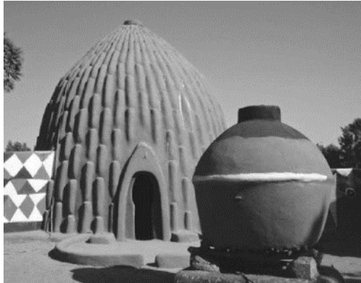
Figure 18: A typical Musgum hut, notice the projected overlapping oval forms that surround the building and served as a ladder for reaching the summit of the hut. The ladders were used for both the construction as well as the maintenance of the structure[2].
