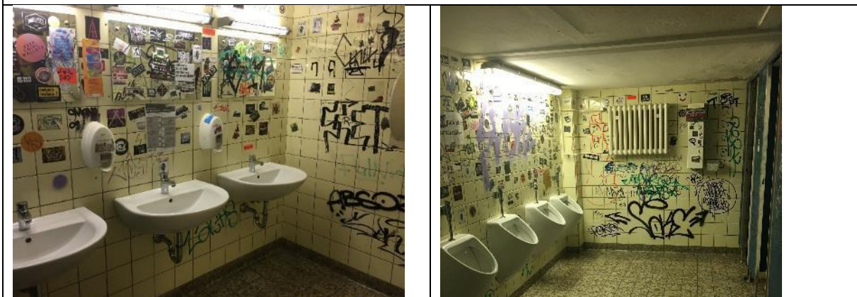
The majority of the toilets are located in the basement, and some are fitted with limited water saving fixtures (relevant for KPIs B2.8 Drainage system design and D3.3 Water saving fixture)
