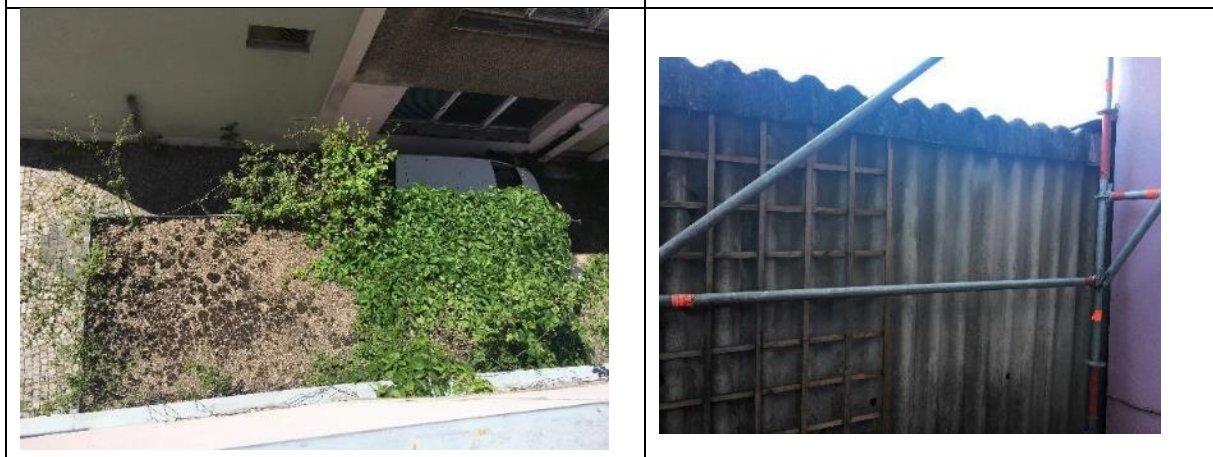
Photos showing the limited outdoor areas of the GAUstrak building, notice the asbestos external fence and the limited space and shading ( relevant for the KPIs B2.12 Site perimeter Slope away from entrances and walking areas, B4.1 Permeable Outdoor Surrounding Surfaces, C1.12 Outdoor shaded area , C1.13 Outdoor area provided with cooling elements such as water features, vegetation or fans, B6.1 Toxin and plastic free outdoor structures and surfaces, and C1.15 Albedo paving surfaces)
