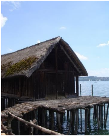
Figure 10: Reconstruction of stone age (4000 B.C) house, located in lake Constance (Germany) showing the building being raised on pillars to adapt water level rise and flooding. Other climate adaptation measures can also be observed.
