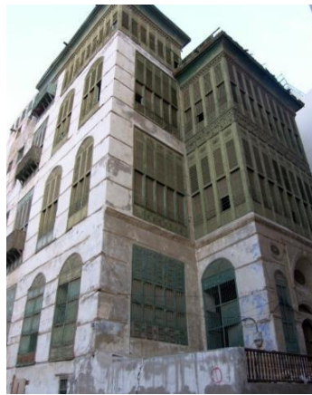
Figure 11: An 18 th century multi generation residential building in the old city of Jeddah (Saudi Arabia). Notice the high multi story wooden covered opening facing Northwest to allow for maximum air circulation and minimize direct solar radiation and glare.
