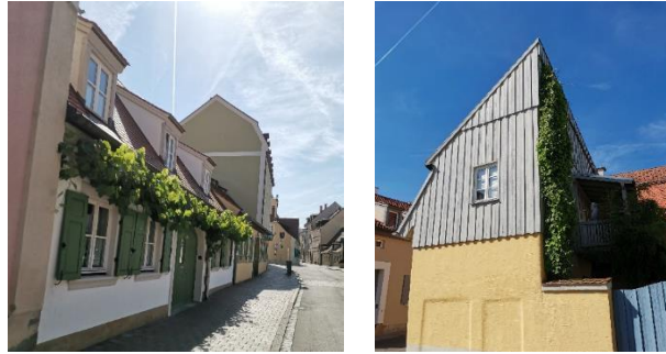
Figure 92: the user of climbing trees over the façade as adaptation solution is common site in Bamberg.
