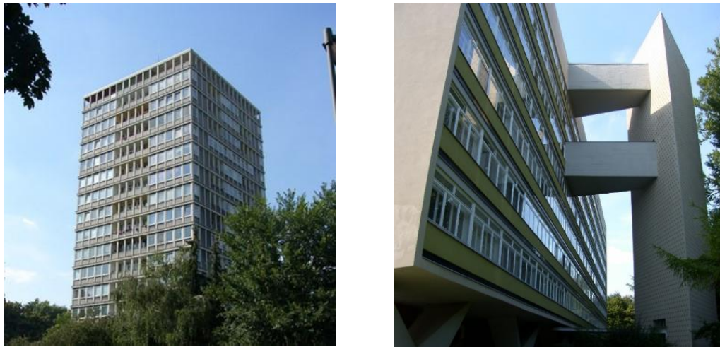
Figure 27 and 28: Examples of 2 nd generation buildings showing extensive use of curtain wall systems and absence of external shading (to the left Bartningallee 9 building by Gustav Hassenpflug) and (image to the right Altonaer Straße 4-14 by Oscar Niemeyer) Both buildings were constructed as part of the Berlin Interbau of 1957
