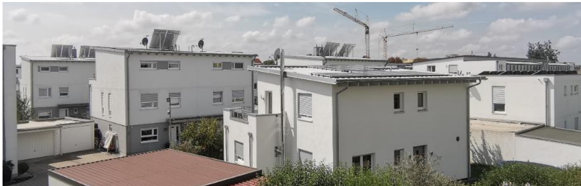
Figure 31: A row residential buildings in Germany built post 2010 showing the typical features of design performance requirements of the 3.0 generation such as the use of solar PVs and solar Collectors on the roof, the relatively small openings, the external solar shading, and the extruded envelope insulation.
