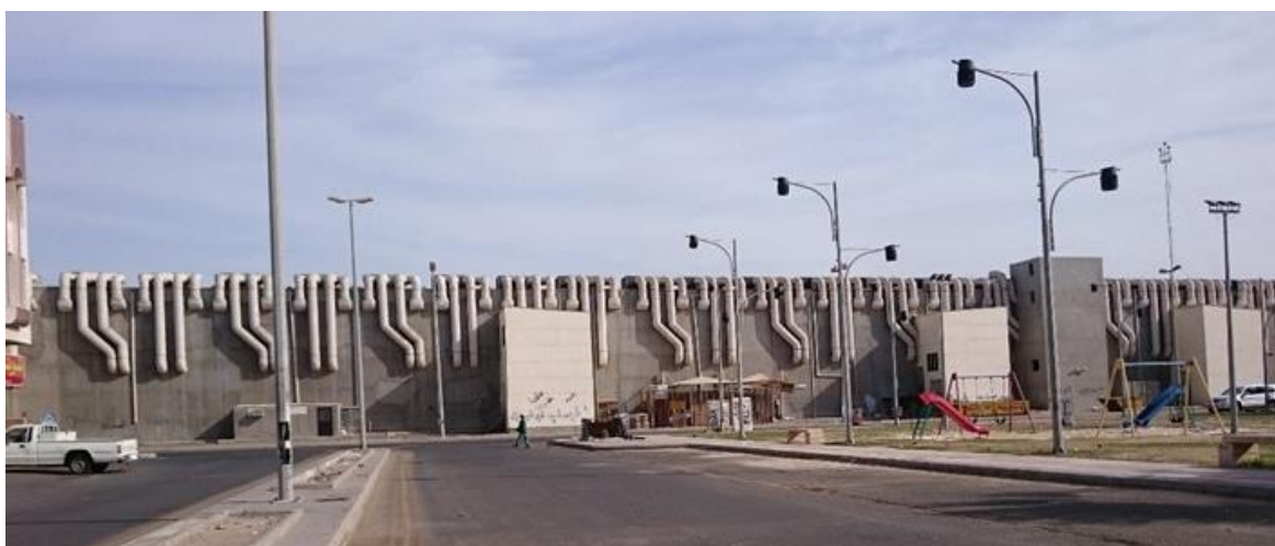
Figure 28: A back alley in Jeddah, Saudi Arabia showing the overreliance on air conditioning and ventilation system that overtook the building back facades.
