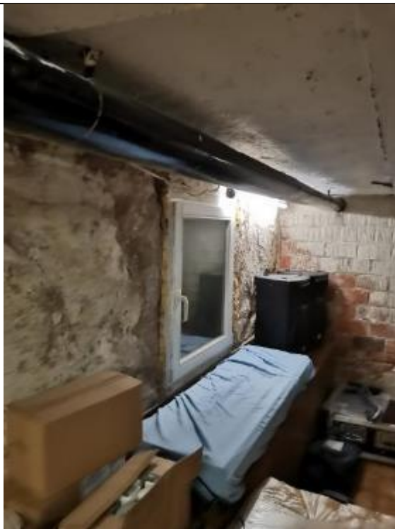
Photos from the technical rooms showing dampness and water leakage damage to the walls (relevant for the KPIB5.2 Leakage and rain proof technical rooms)
