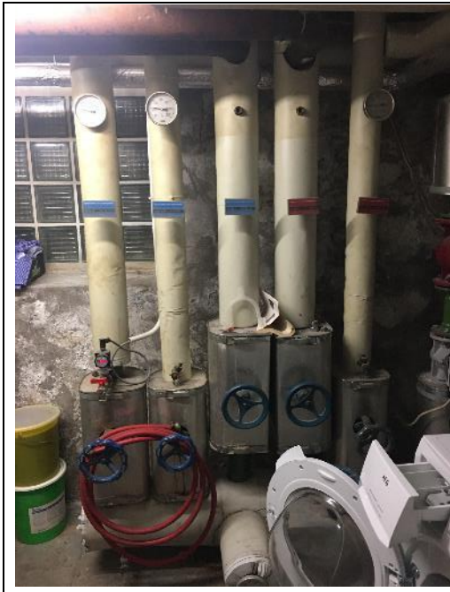
Photos showing the cramped situation of the technical pathways and limited access to the technical rooms (relevant to the KPIs B5.3 Protected and diverse technical pathways and B5.4 Ease of access, maintenance of technical systems and rooms)
