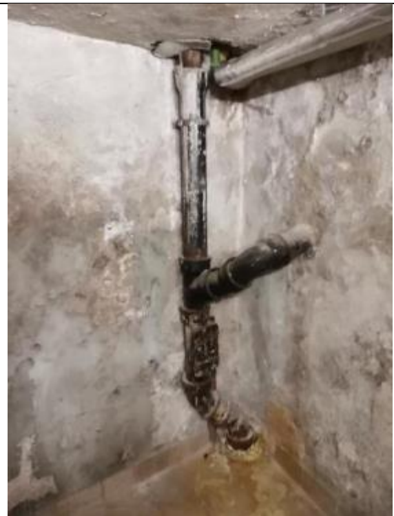
Photos from the technical rooms showing dampness and water leakage damage to the walls (relevant for the KPIB5.2 Leakage and rain proof technical rooms)
