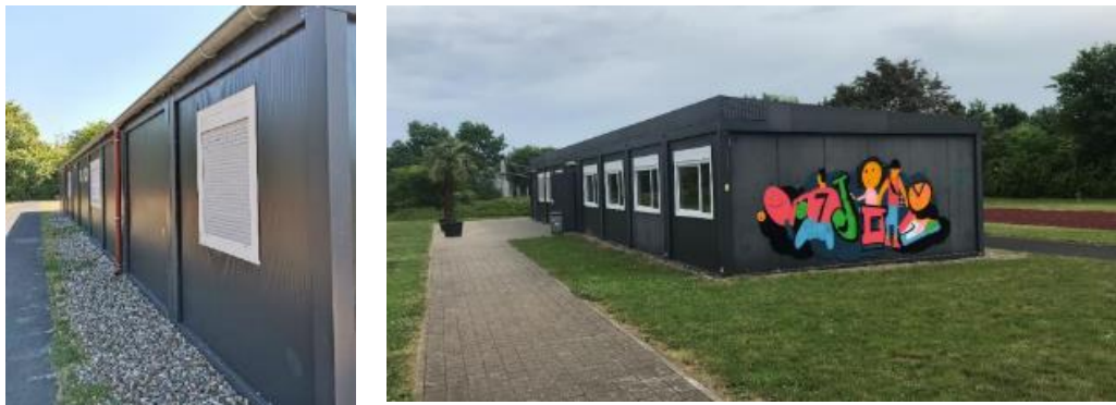
Figure 65: A frontal and back images of the JO container building
