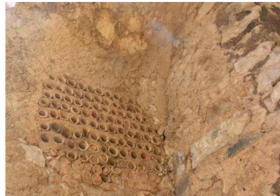
Figure 23: Clay ventilation ducts used by the Roman engineers to cool the subterranean domus in ancient city of Bulla Regia in present day Tunisia.
