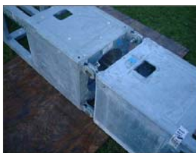
Abb. 4-16. Maststoss (44)
