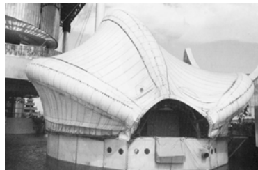
Abb. 3-84. Electric Power, Osaka (14)
