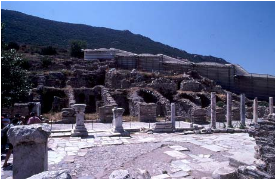
Figure 6.11 The protective shelter of the Terrace Slope Houses 2 aims to protect the valuable material against climatic and environmental conditions as well as intensive visitation. The visual harmony of the modern structure with the archaeological landscape and topography is debatable.
