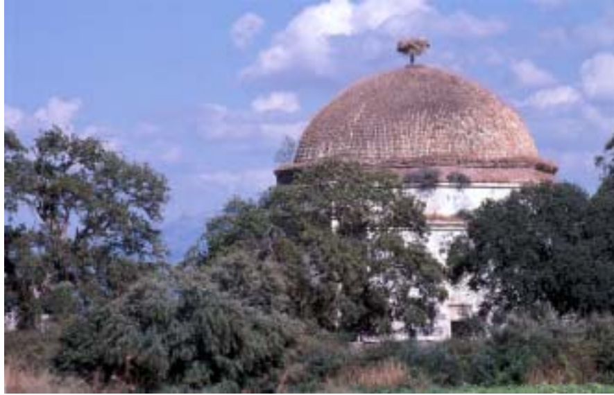
Figure 4.7 The İlyas Bey Mosque built in 1411-1416 A.D. at the archaeological site of Miletos. Beside the ancient structures, buildings from Ottomans embedded in the landscape can be also seen at Miletos.
