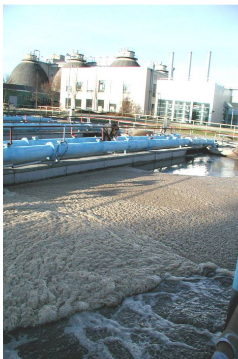
Figure 1: Stable scum layer floating on the aeration tank (C-elimination and pre-denitrification) of a municipal WWTP.
