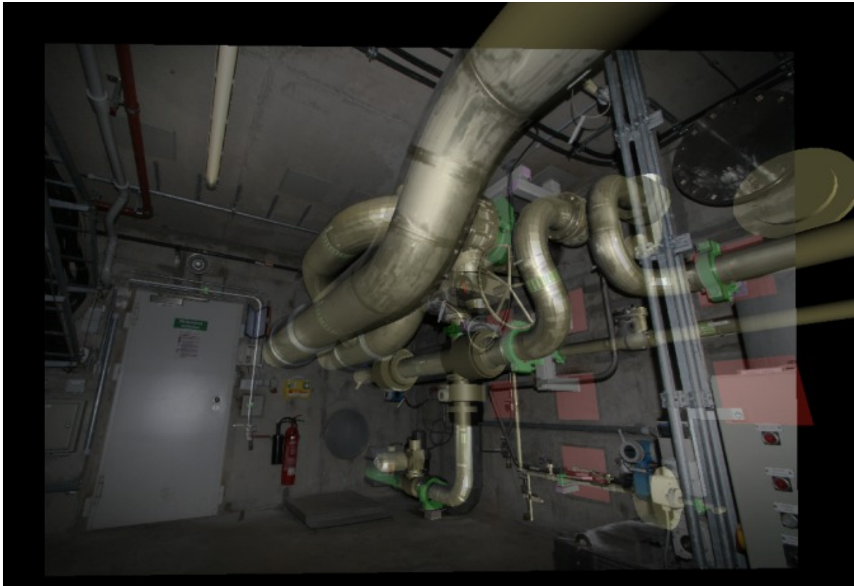
Figure 4.4: VID an augmented CAD viewer: VID supports the inspection of CAD Model via augmented reality. It offers to align and display an image within a CAD Model.
