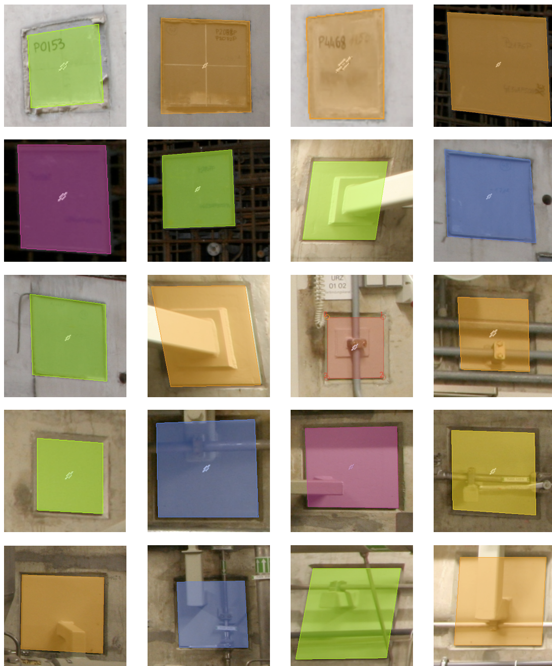
Figure 6.2: Results of Anchor-Plate Segmentation. These segmentations were obtained using a region of interest around the anchor-plates and were always within the ten first candidates proposed by the algorithm.
