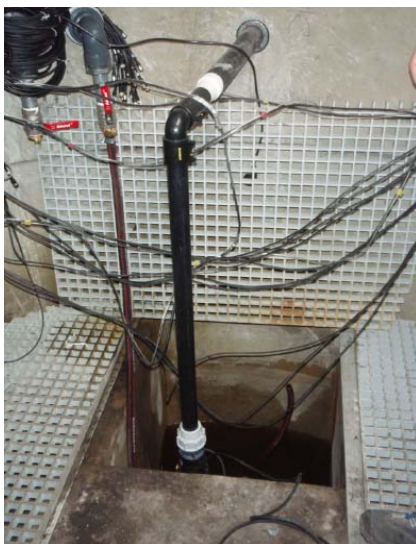
Abb. A3.26: Pumpensumpf
