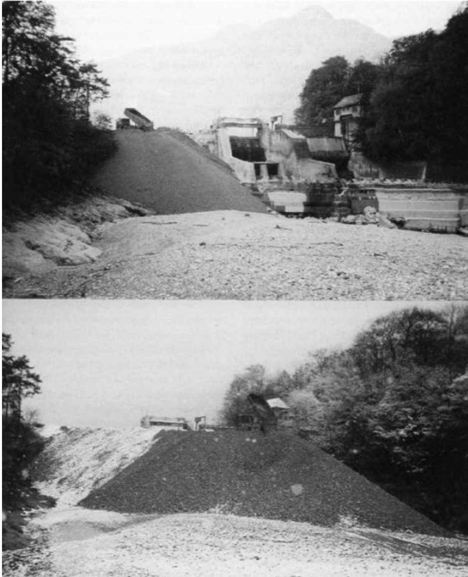
Fig. 1.5 Supply of fine material downstream of Kiblinger Sperre (River Saalach) (Courtesy of LfU, Schaipp)
