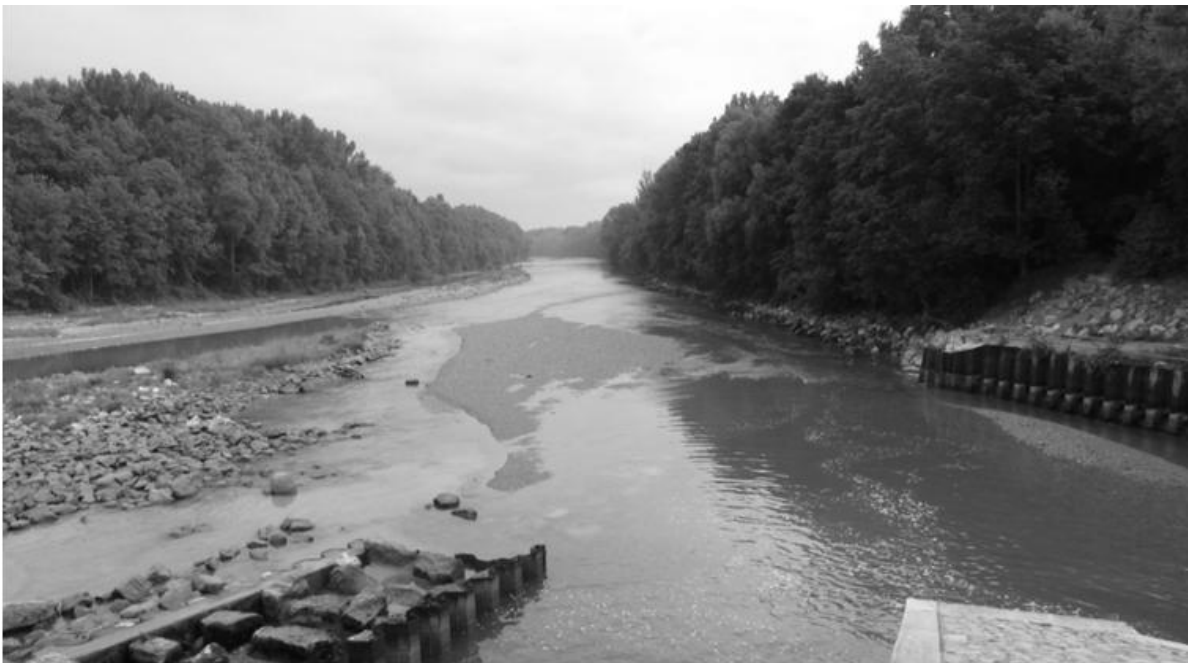
Fig. 1.4 Bed surface downstream of Eisenbahnerwehr after flushing activity
