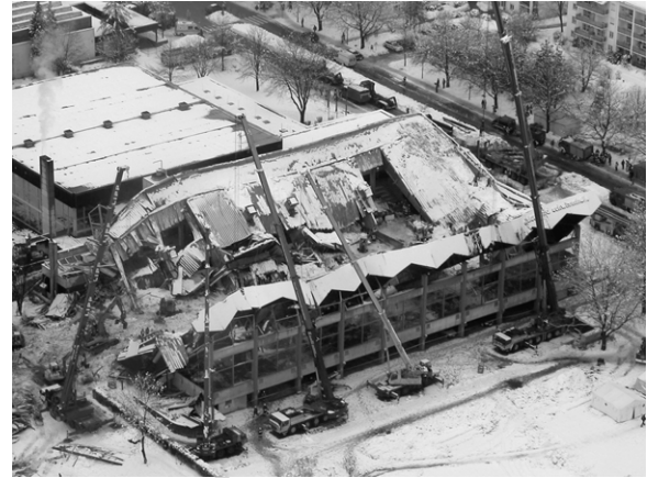
Fig. 7. Top view on Bad Reichenhall Ice-Arena after progressive collapse of all main girders (Photo: LKA Bayern).
