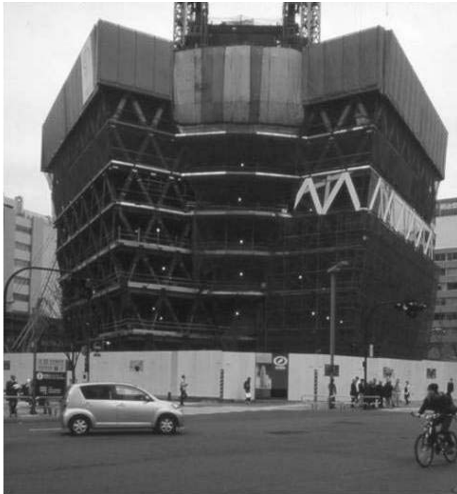
Self-climbing cover and scaffolding structure partly structuring the assembly environment on-site
