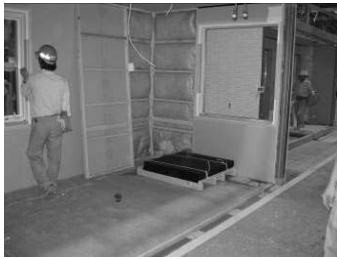
Quality control interior
