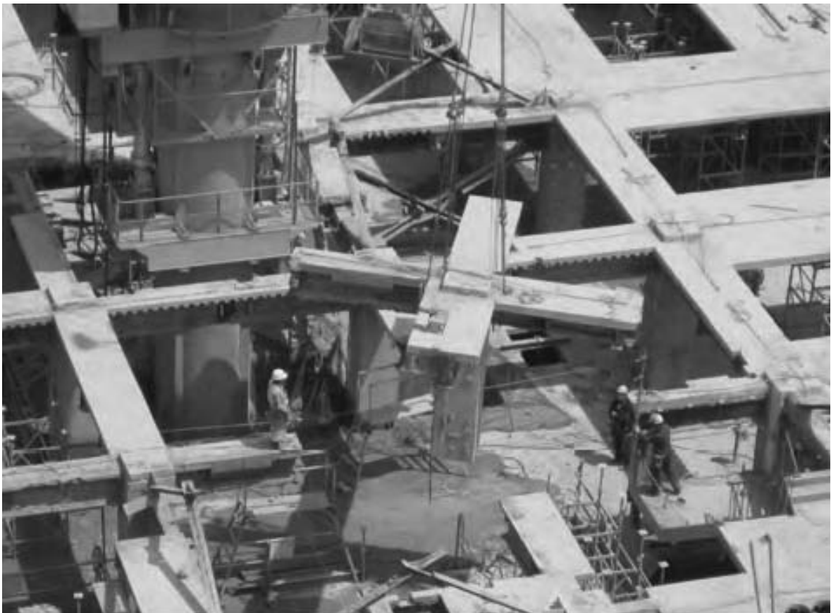
Cutting off and picking up of component in OSF (RIBC, 2012)
