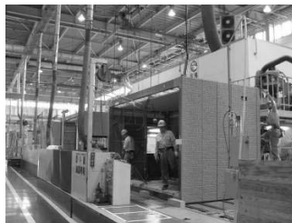
Assisted placing of insulation
