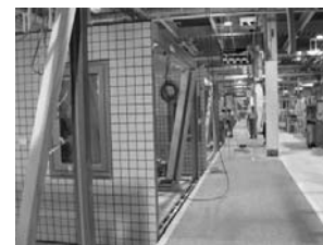
Step-by-step cabling on production line
