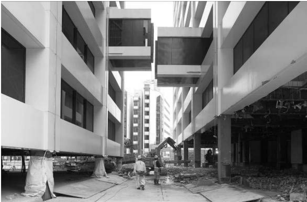
On ground disassembly of lowered and prepared floors (Kajima, 2009)
