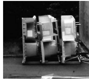
Equipping of bottom plates with technical installation
