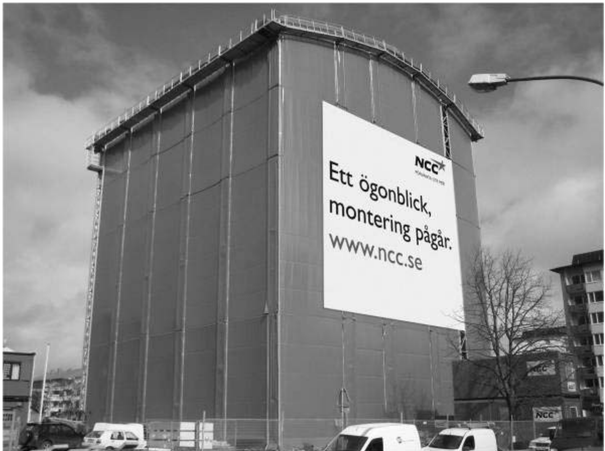
On-site factory (NCC, 2012)
