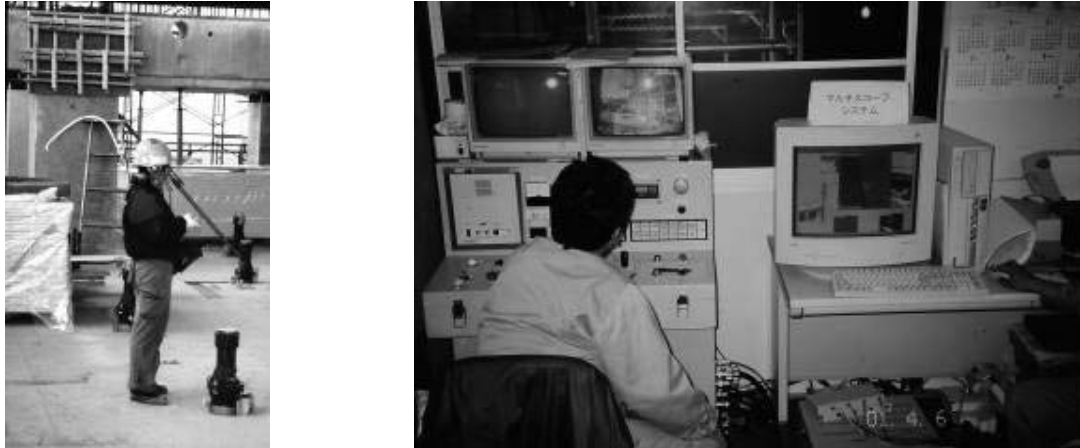
Figure 7-1: Left: female worker on the construction site remote controlling and supervising the operation of ABCS subsystems. Right: Worker in control room supervising processes and construction progress.
