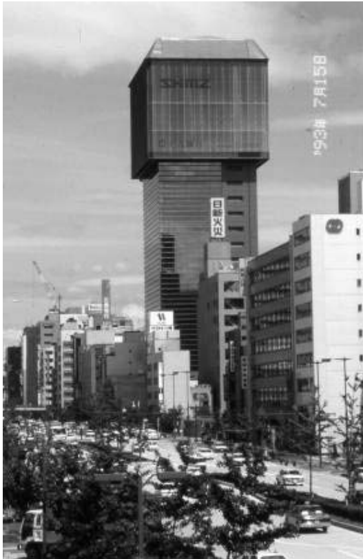
Figure 2-12: Shimizu's SMART is a modular automated on-site factory with modular robotic (overhead) manipulators and modular exchangeable end-effectors. Apart from the flexibility allowed by modularity, the manipulators and the end-effectors integrate in-built flexibility (for example, through re-programmability)
