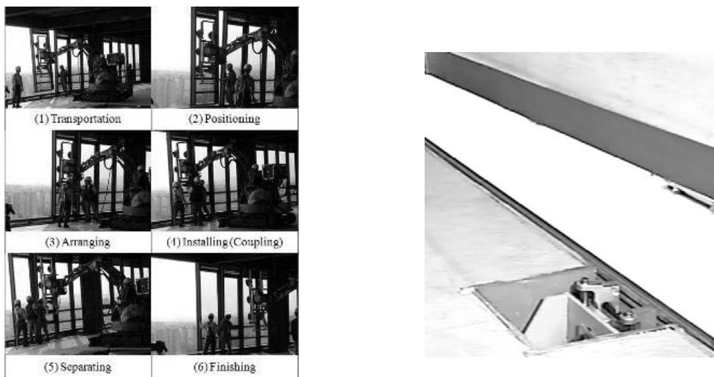
Figure 6-12: Reduction of organizational complexity. Left: A Korean facade installation robot requires three workers to be operated and does thus not fulfill the requirements to reduce organizational complexity (picture courtesy of Lee, see also Lee, 2008 ). Right: ABCS uses connectors in combination with a robotic overhead crane, reducing the number of workers to only one worker supervising many parallel activities at once, and the need for assisting workers guiding the component has been completely removed (graphical representation according to Obayashi, 1993 )
