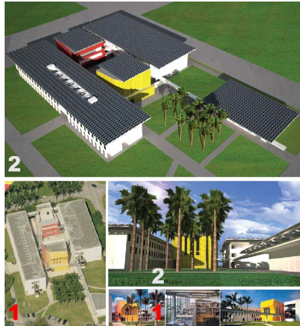
Figure 8: Images 1 show the existing PCA complex. Images 2 show the Net-Zero-PCA simulation with the new building integrated 5,388 m 2 (58,000 sf) Sun Power PV arrays. Source: Author, 2013.
