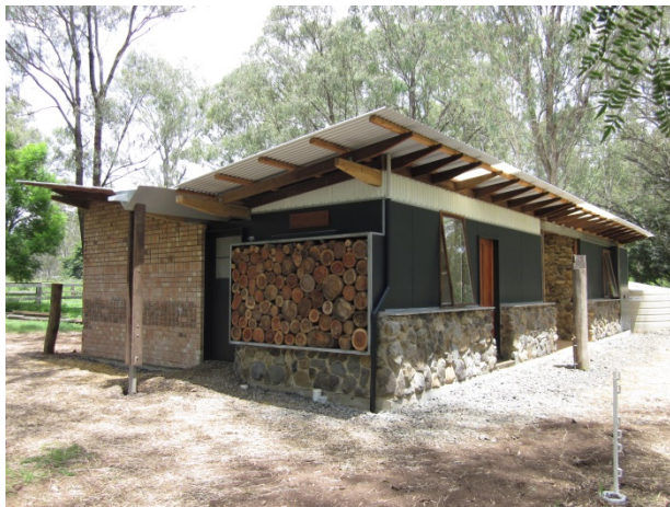
Figure 3. The finished building showing deviations from the original design through material-induced design changes
