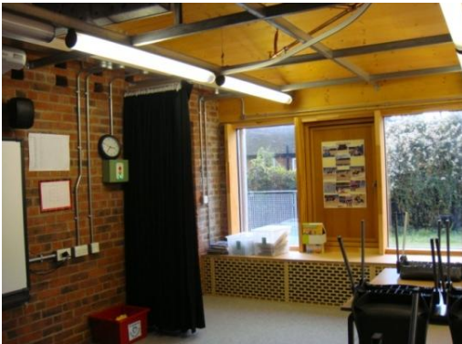
Figure 7: Exposed masonry wall, lighting and air intakes underneath windows in a classroom, School B.
